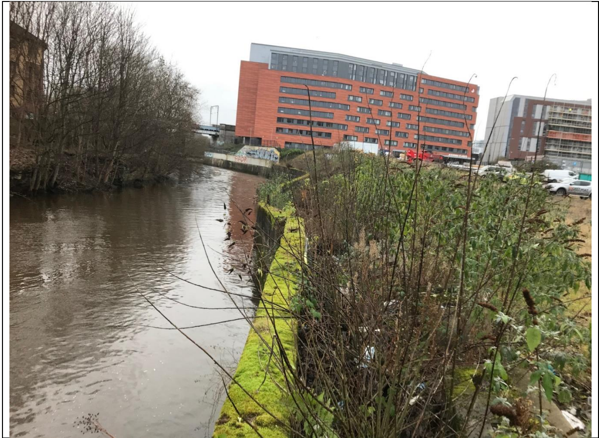
Site looking West , along top of quay wall.
