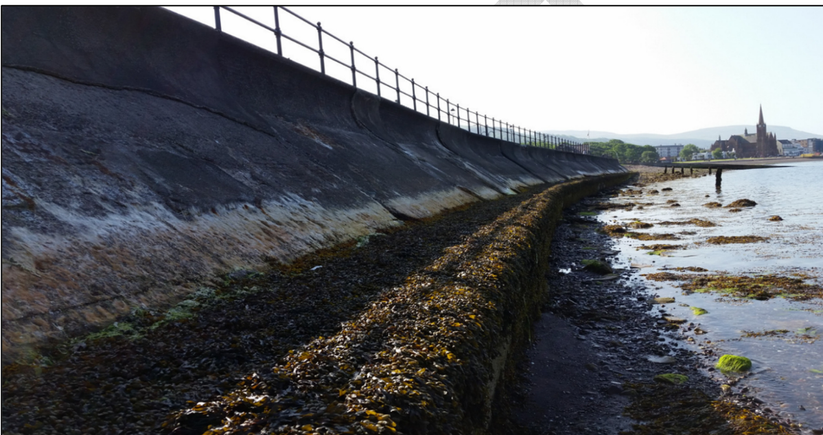
Figure 3: Southern end of the Existing Seawall
