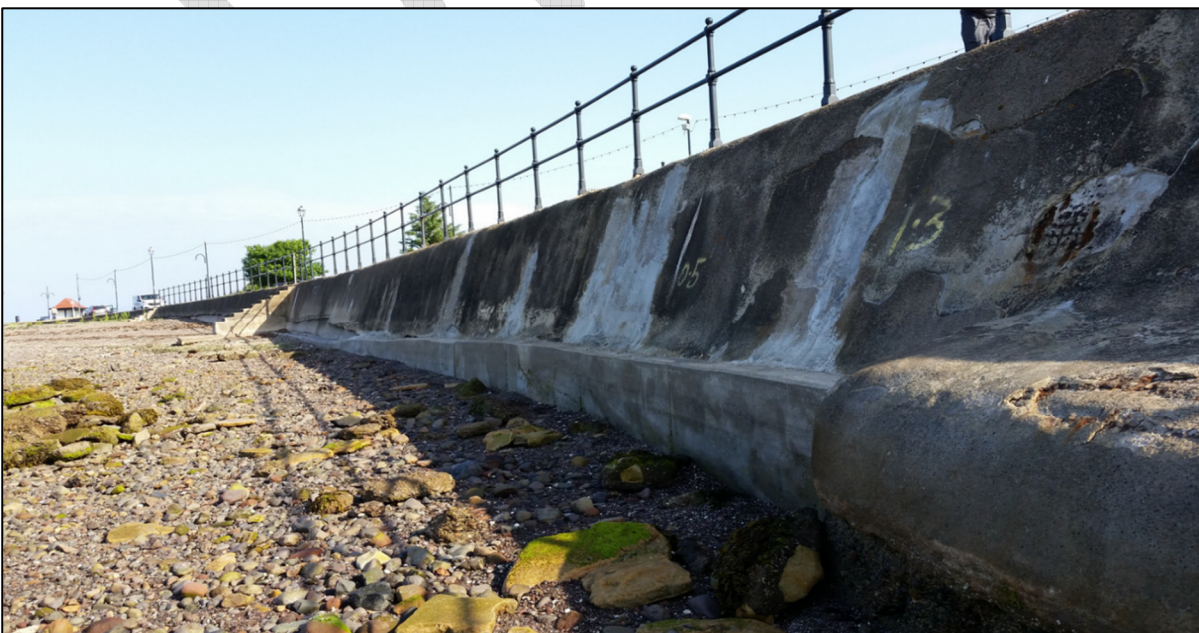
Figure 4: Northern end of the Existing Seawall
