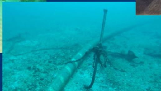
Subsea Cable subject to damage
