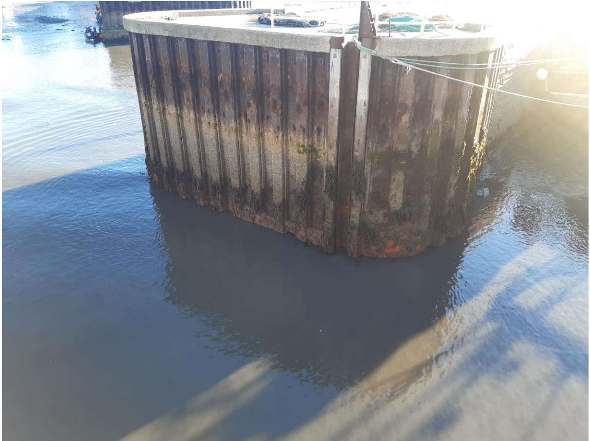
South Pier – Typical Condition
