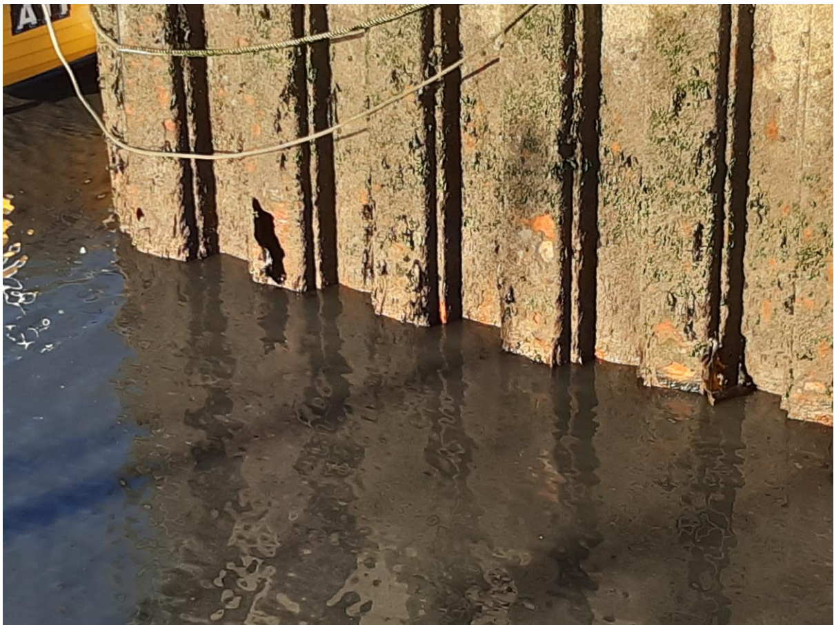
Fish Jetty – Typical Condition
