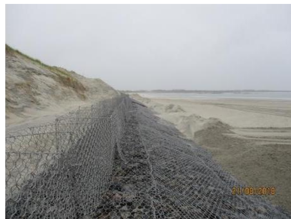
Fig 3. A typical representation of the sloping Reno mattress and top edge basket on a graded sand dune
