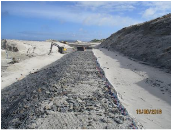
Fig 4. A view from atop a completed mattress installation prior to the dune face being reinstated
