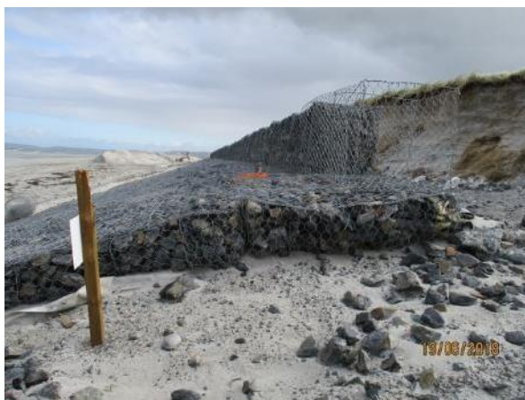
Fig 2. A cross sectional view of the Reno Mattress and gabion basket configuration
