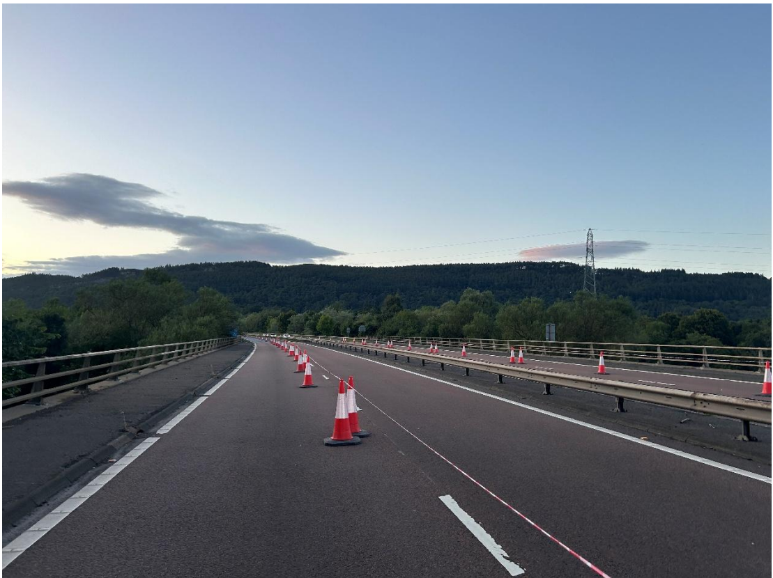
Figure 3. Typical view of the carriageway and bridge facing north.
