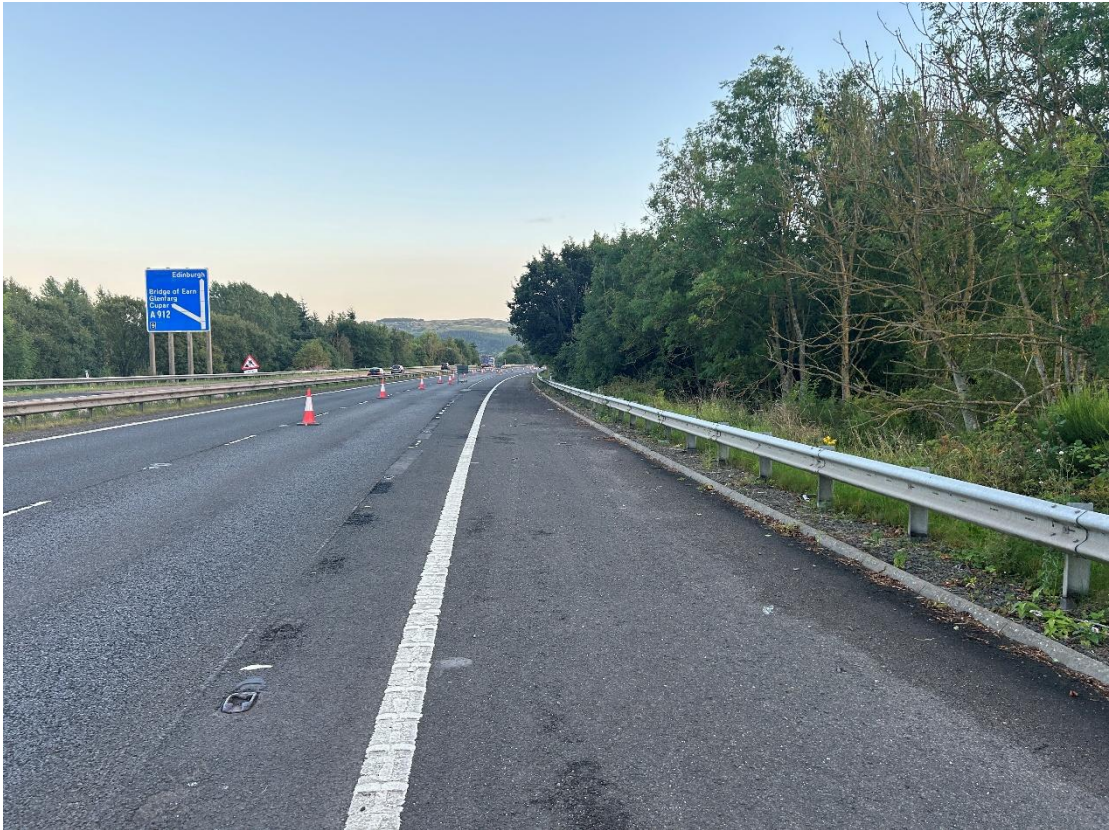
Figure 2. Typical view of the carriageway and structure facing south.
