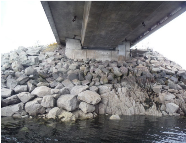
Figure 5, A87 Carrich Bridge – Typical view from underneath the bridge of the concrete box girder soffit, rock armour, abutment and water main.
