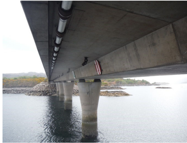
Figure 6, A87 Carrich Bridge – Typical view of the box girder soffit, water main, drainage gullies, water main and daymark boards and bridge deck cantilever.
