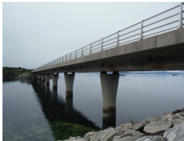
Figure 4, A87 Carrich Bridge – Typical view of the bridge piers, concrete box girder and parapet from below the bridge.
