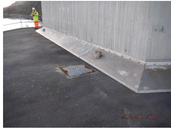
Figure 10, A87 Skye Bridge – Typical view from on Pier 3 & 4 of the bentonite cover.
