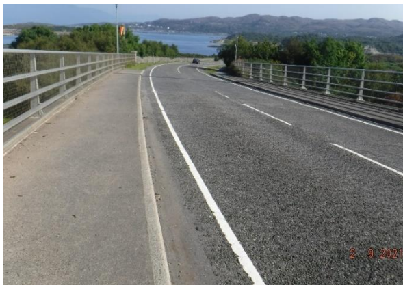
Figure 7, A87 Skye Bridge – Typical view of carriageway and footpaths.
