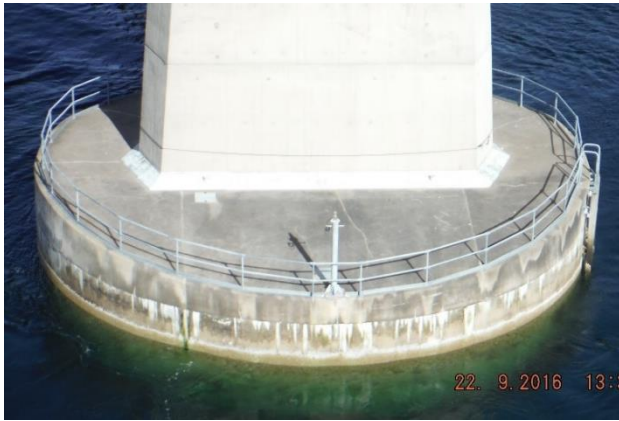
Figure 9, A87 Skye Bridge – Typical view of one of the main pier caissons and bentonite covers (Piers 3 & 4) within the tidal Channel of Loch Alsh.
