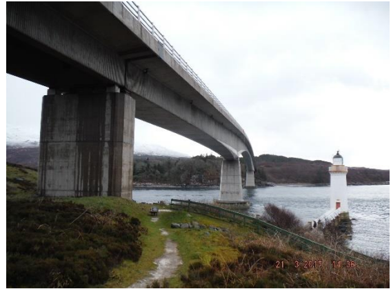
Figure 4, A87 Skye Bridge – Typical view from Eilean Bàn.
