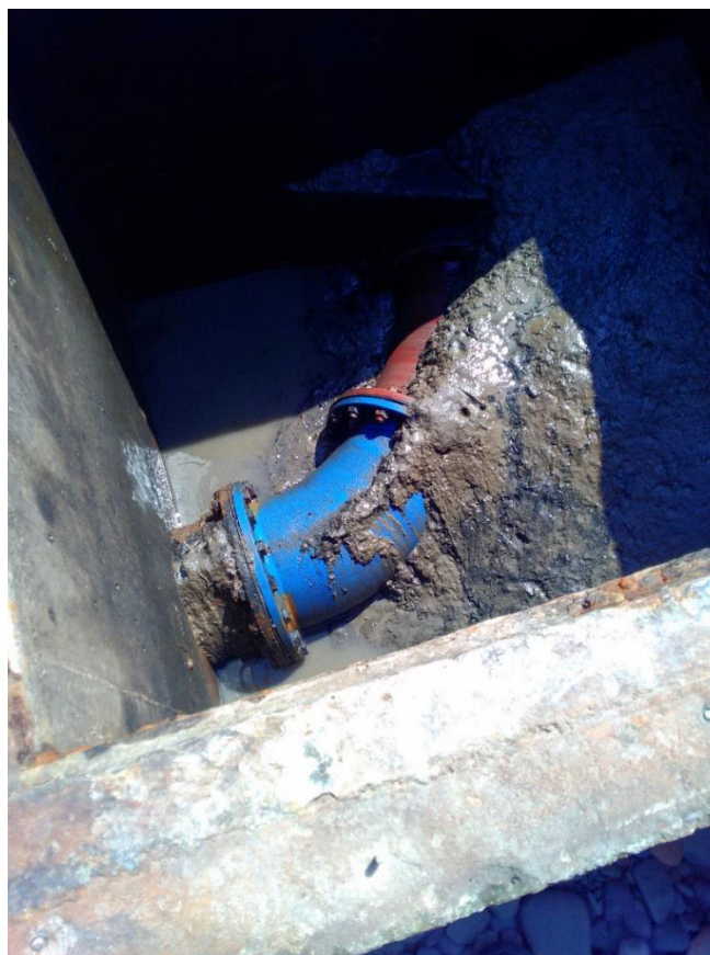
Figure 9 Elbows joints inside inspection chamber (Macfarlan Smith).
