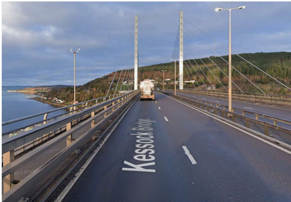
Existing redundant anemometer on west (left) side of the Bridge North-east Pylon is on the right of the picture
