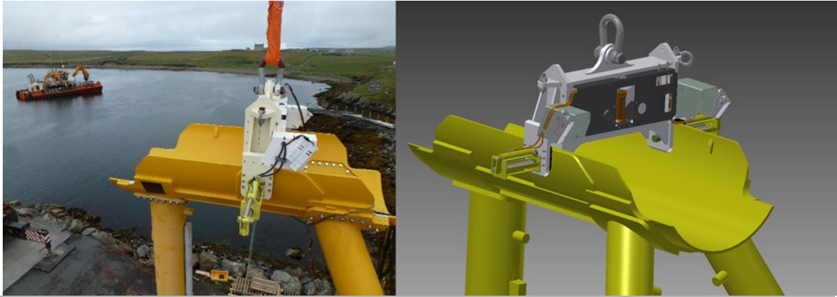
Figure 5-2: Universal lifting tool used for lifting fully ballasted turbine substructures.
