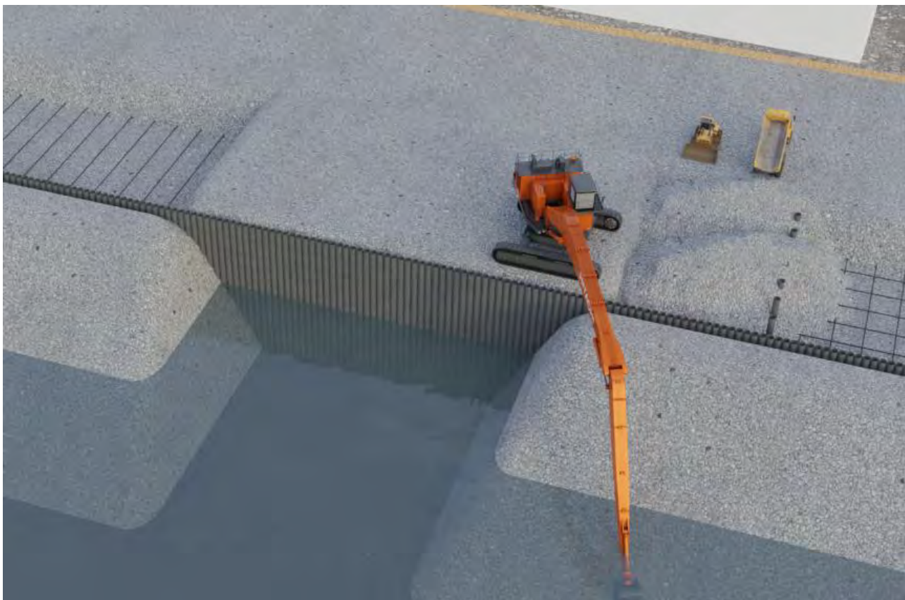
Removal of Temporary Stone Bund
