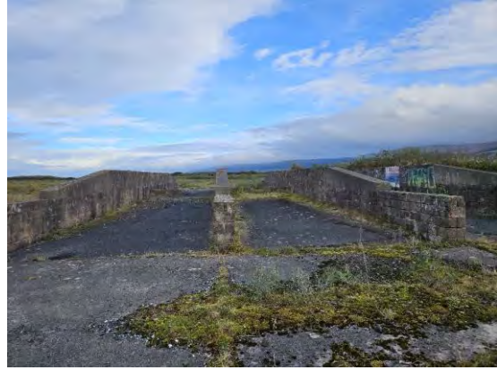
Photo 8: Walls on site.
