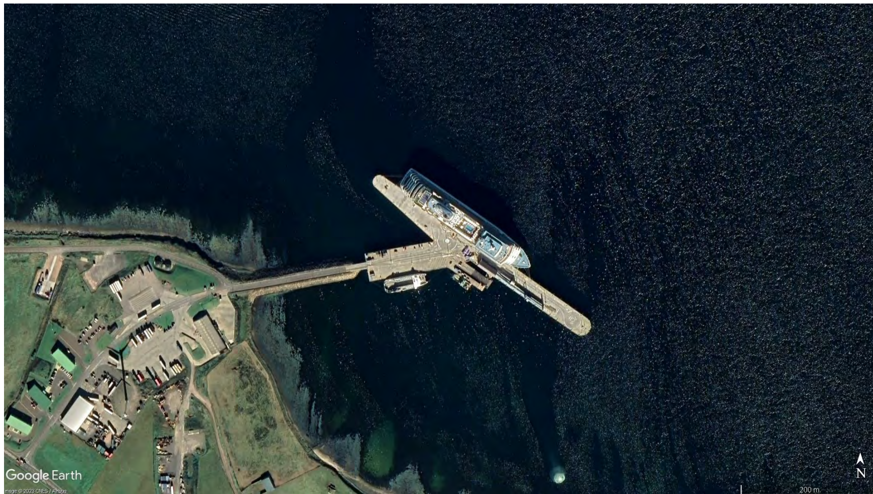
Figure 2-3: Satellite image of existing Hatston pier structure
