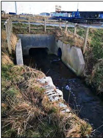
Photograph 1: Culverted entrance to Burn of Hatston, with limited fish suitability
