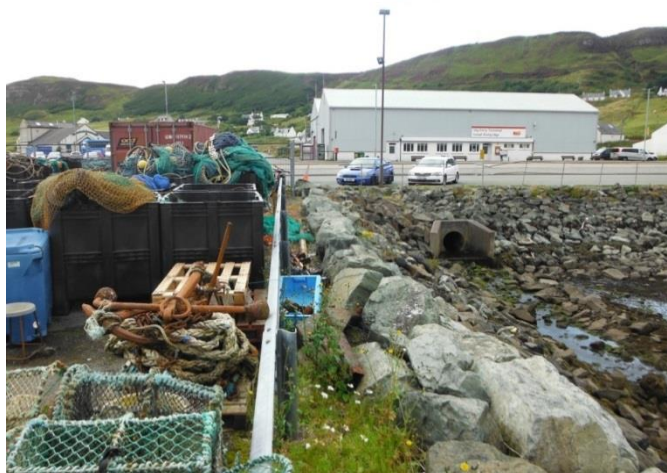
Photograph 9-2 Culvert Overflow of Small Watercourse
