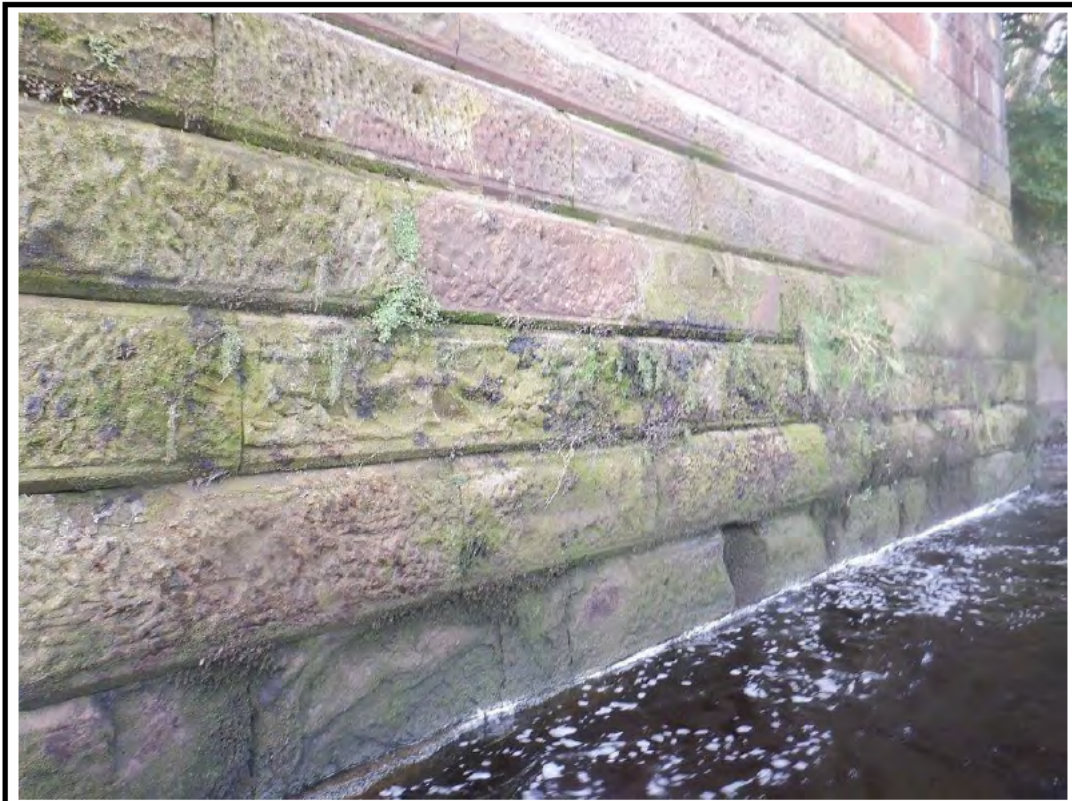
PHOTO 20: P20 - PIER 1 ANNAN STATION (HIGH MILEAGE) FACE 14/09/20
