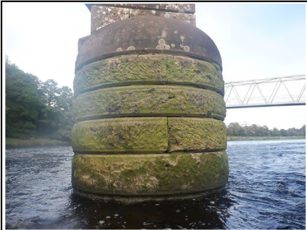
PHOTO 26: P26 - PIER 3 DOWNSTREAM NOSE 14/09/20
