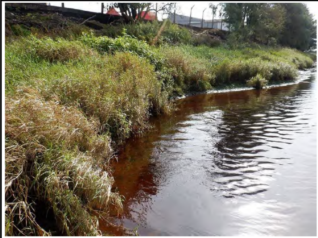
PHOTO 11: P11 - EROSION DOWNSTREAM HIGH MILEAGE 14/09/20
