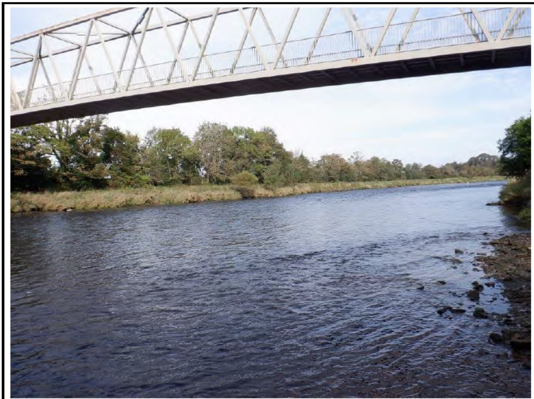
PHOTO 2: VIEW LOOKING UPSTREAM FROM STRUCTURE 14/09/20
