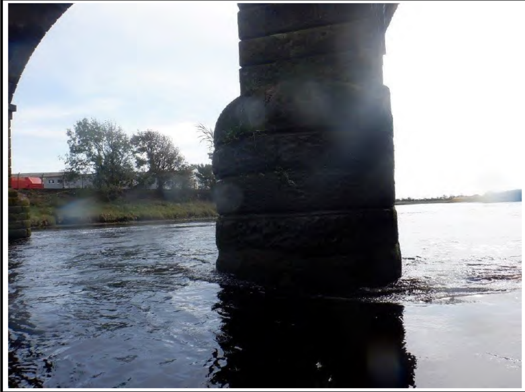
PHOTO 23: P23 - PIER 2 UPSTREAM NOSE 14/09/20
