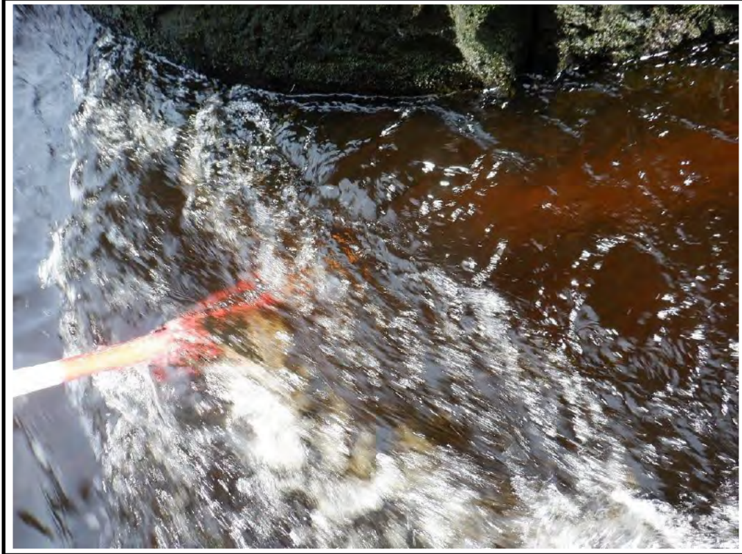
PHOTO 5: P5 - DAMAGED GABIONS 14/09/20
