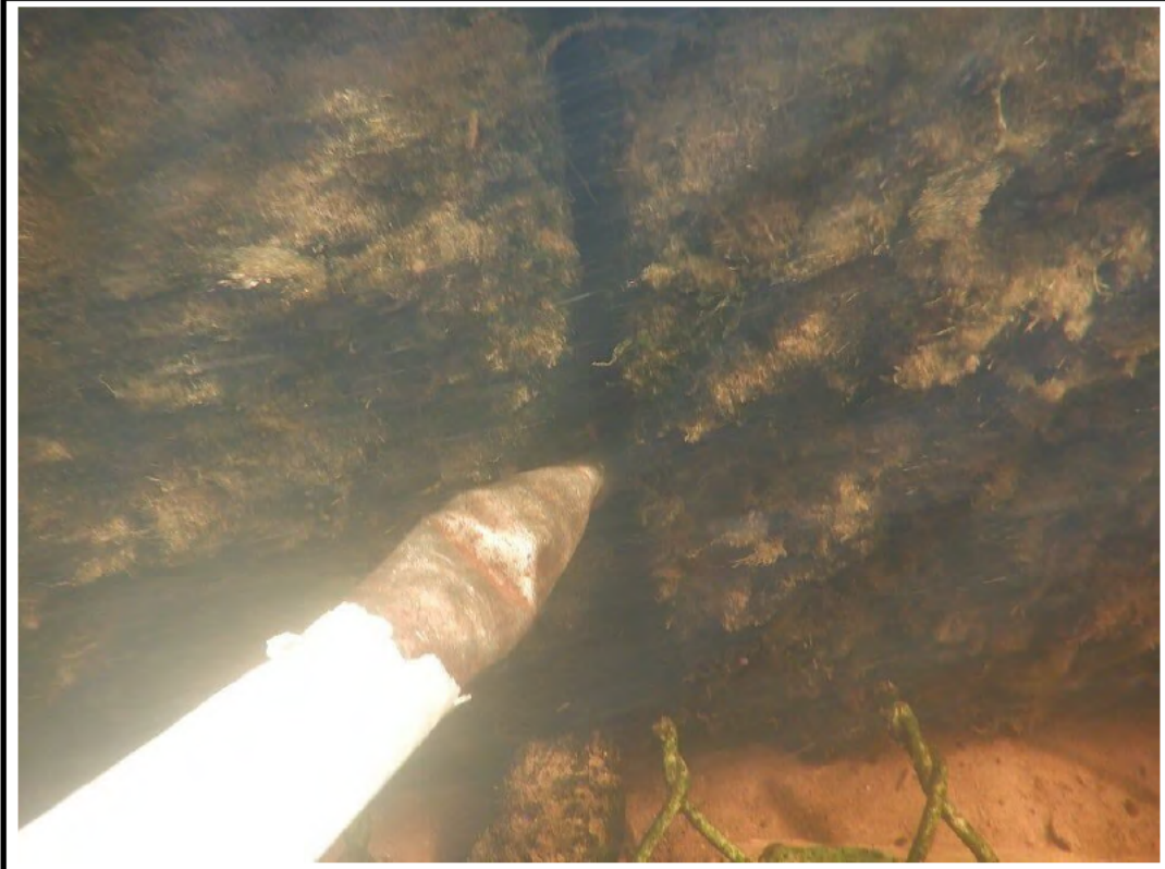
PHOTO 33: P33 - PIER 4 LM FACE 14/09/20
