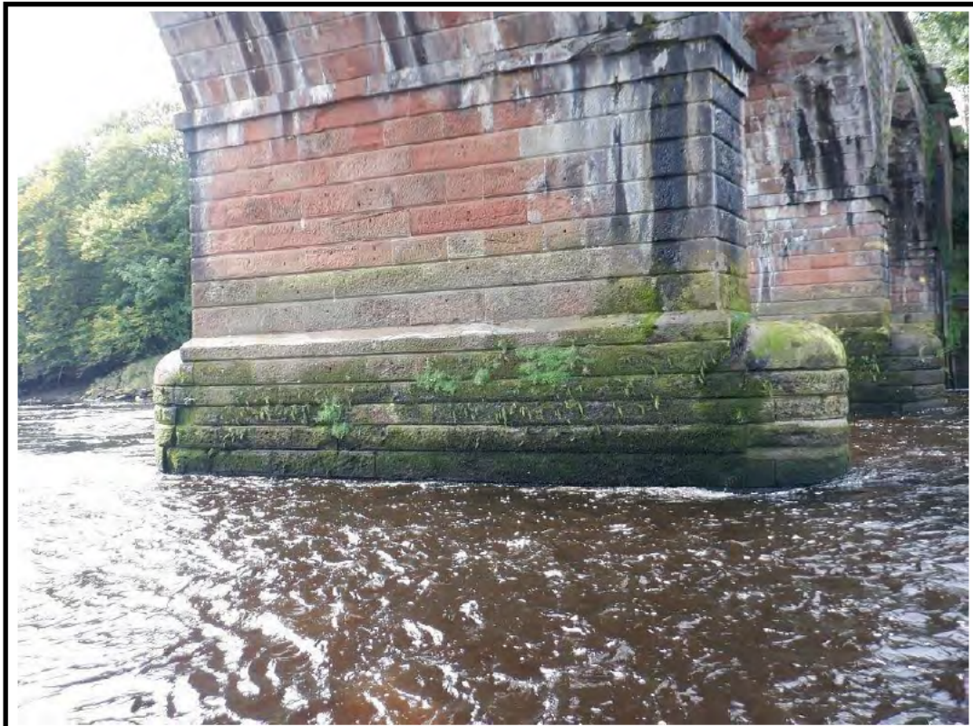
PHOTO 30: P30 - PIER 3 HM FACE 14/09/20
