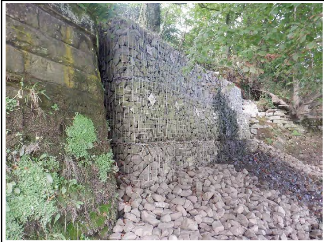
PHOTO 19: P19 - UPSTREAM GABION BASKETS PROTECTED BY PITCHING STONE 14/09/20
