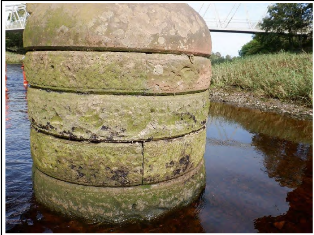
PHOTO 31: P31 - PIER 4 DOWNSTREAM NOSE 14/09/20
