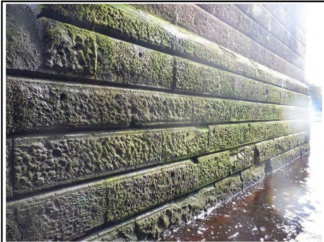
PHOTO 24: P24 - PIER 2 LM FACE 14/09/20
