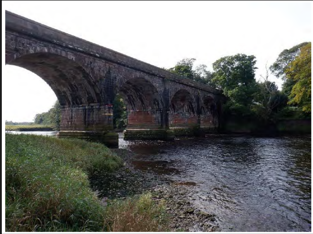
PHOTO 1: VIEW FROM UPSTREAM 14/09/20
