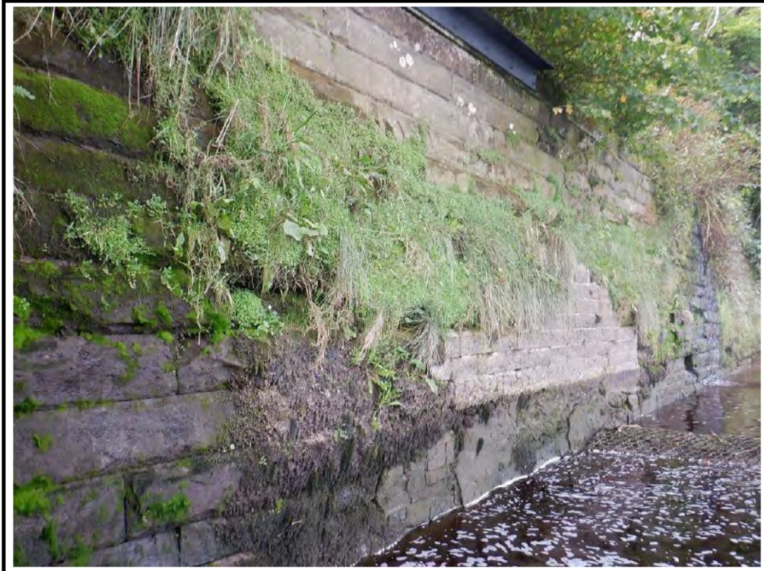
PHOTO 15: P15 - UPSTREAM LM RETAINING WALL 14/09/20
