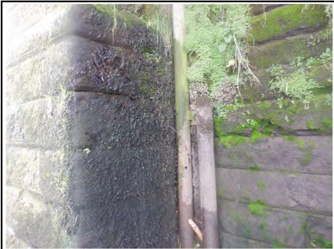
PHOTO 16: P16 - DOWN PIPES LOCATED ADJACENT TO THE ABUTMENT 14/09/20
