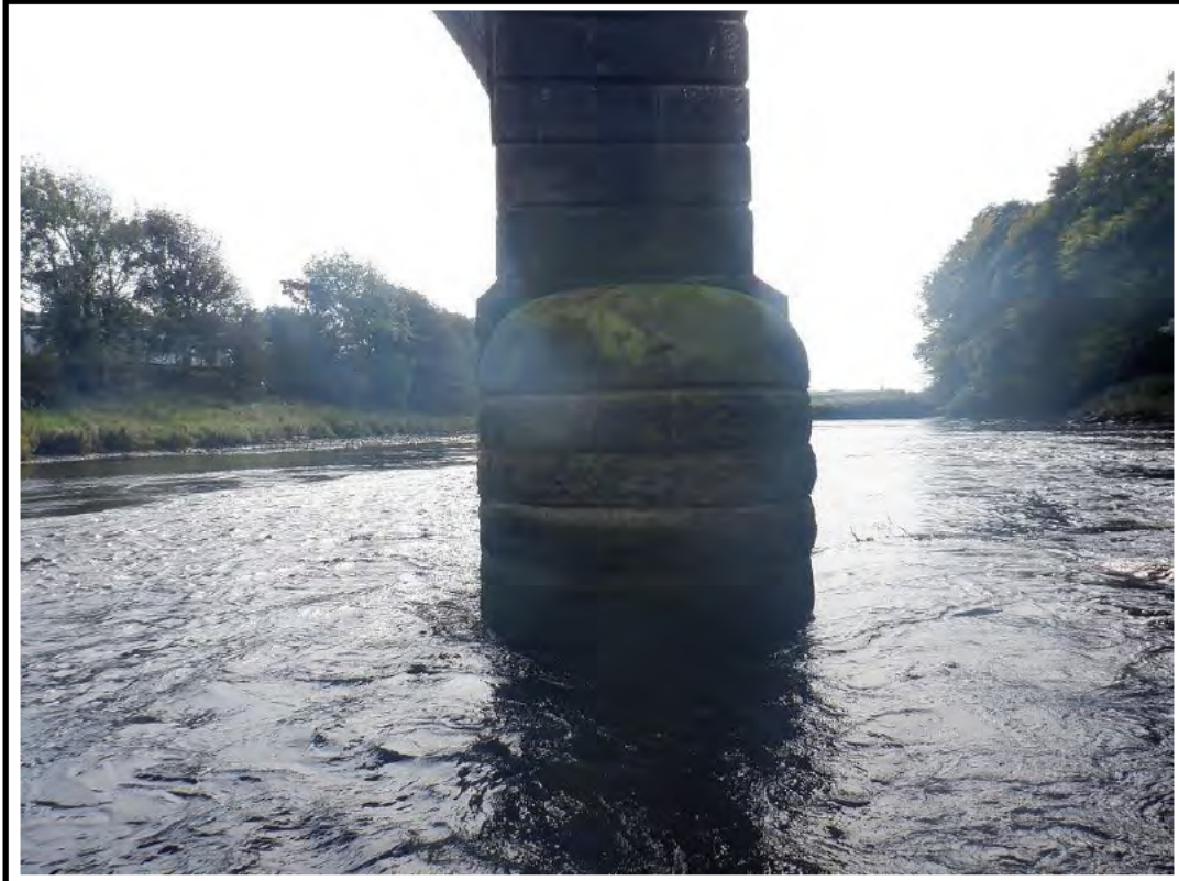
PHOTO 27: P27 - PIER 3 UPSTREAM NOSE 14/09/20
