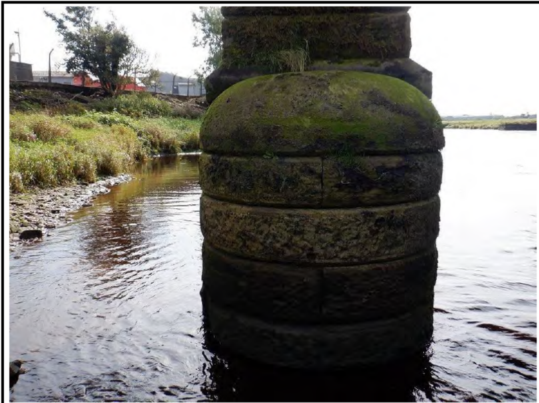
PHOTO 32: P32 - PIER 4 UPSTREAM NOSE 14/09/20
