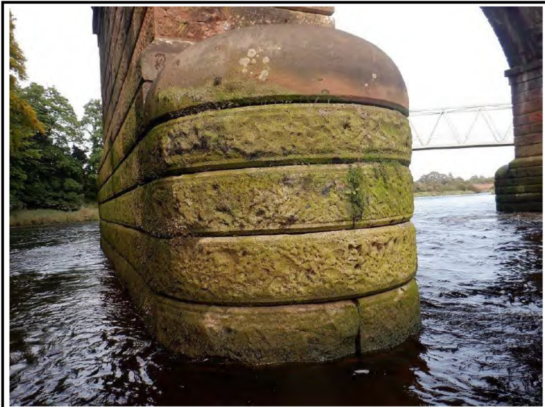
PHOTO 22: P22 - PIER 2 DOWNSTREAM NOSE 14/09/20
