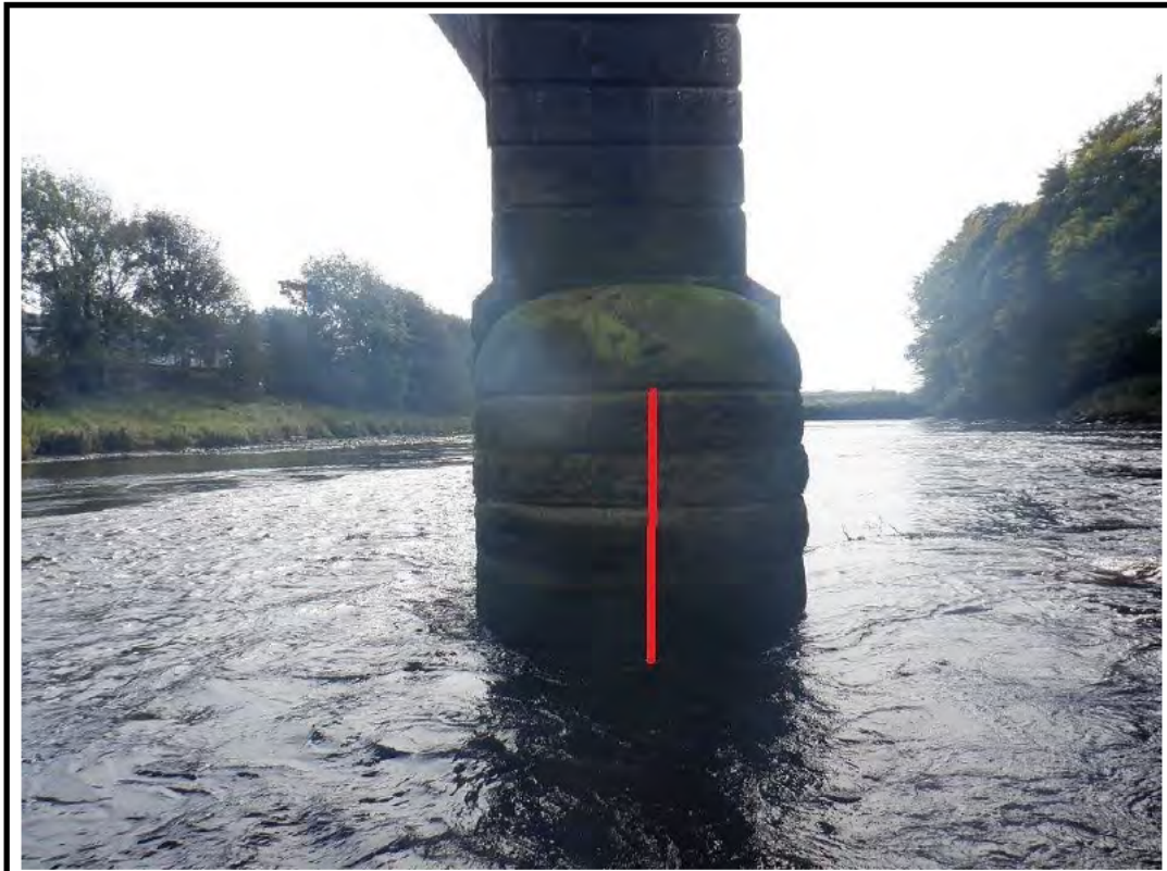
PHOTO 36: P36 - DATUM - PIER 3 UPSTREAM NOSE 14/09/20
