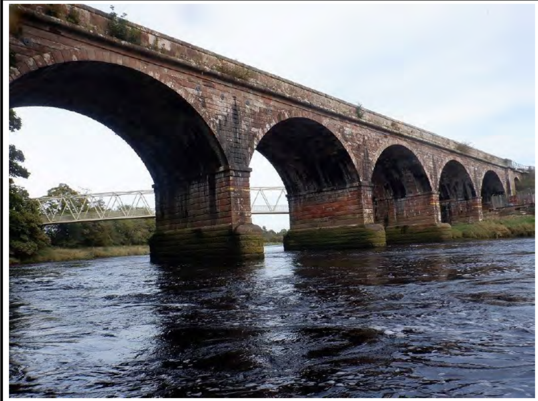
PHOTO 3: VIEW FROM DOWNSTREAM 14/09/20
