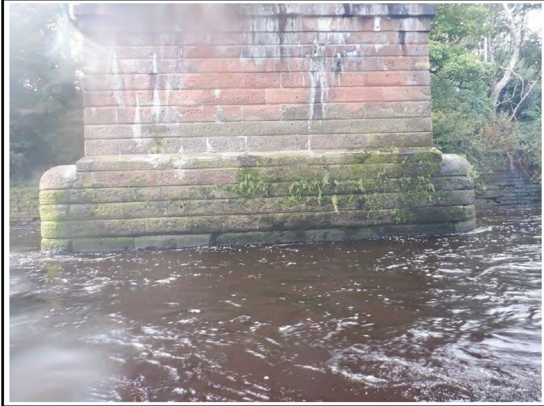
PHOTO 25: P25 - PIER 2 HM FACE 14/09/20
