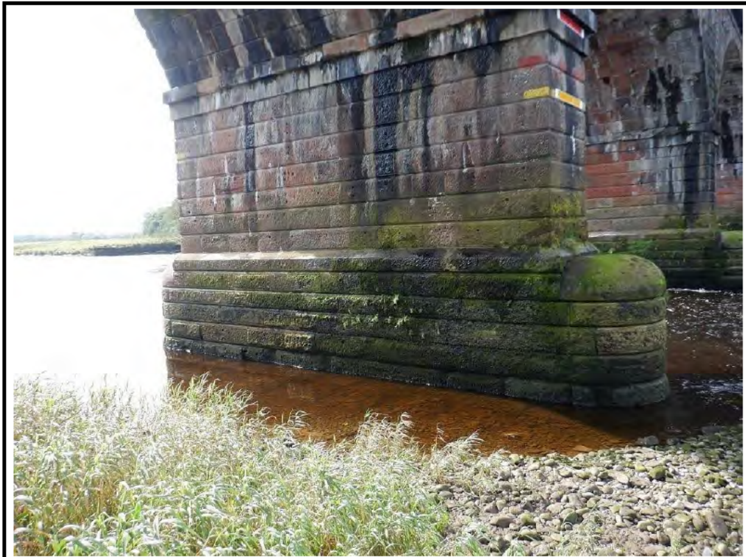
PHOTO 34: P34 - PIER 4 HM FACE 14/09/20
