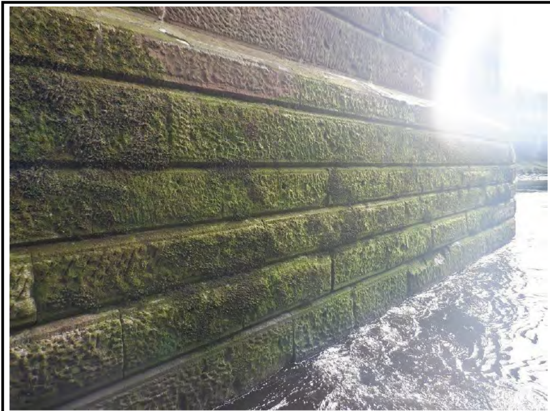
PHOTO 28: P28 - PIER 3 LM FACE 14/09/20
