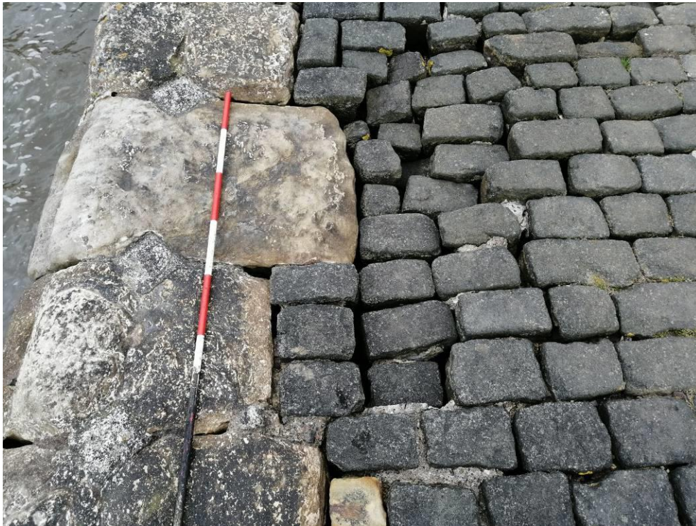
Photo 30 - Example of poor condition sets typical behind cope stones along eastern slipway (image top is south aligned). Red and white increments on staff at 200mm intervals.
