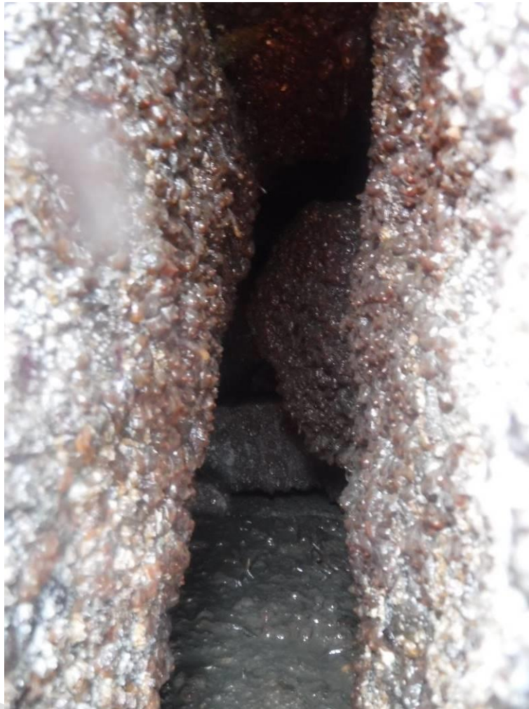
Photo 13 – Close up of crack in western end of north pier outer wall. Note rounded cobble sized material visible behind dressed facing stone.
