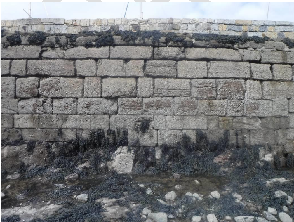
Photo 23 – Water seepage observed from wall interface with possible bedrock at toe of structure. Note dilated joints visible in upper wall stonework.
