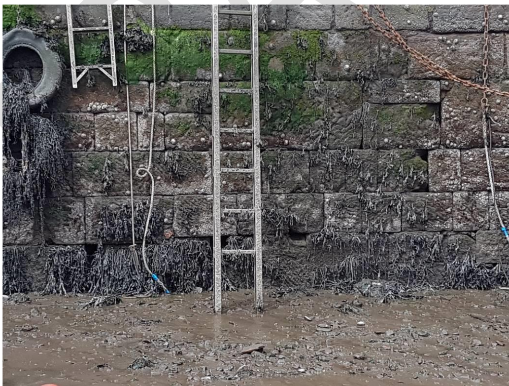
Photo 15 – View of typical stone work within inner wall of west pier, note missing mortar and minor voids between blocks.
