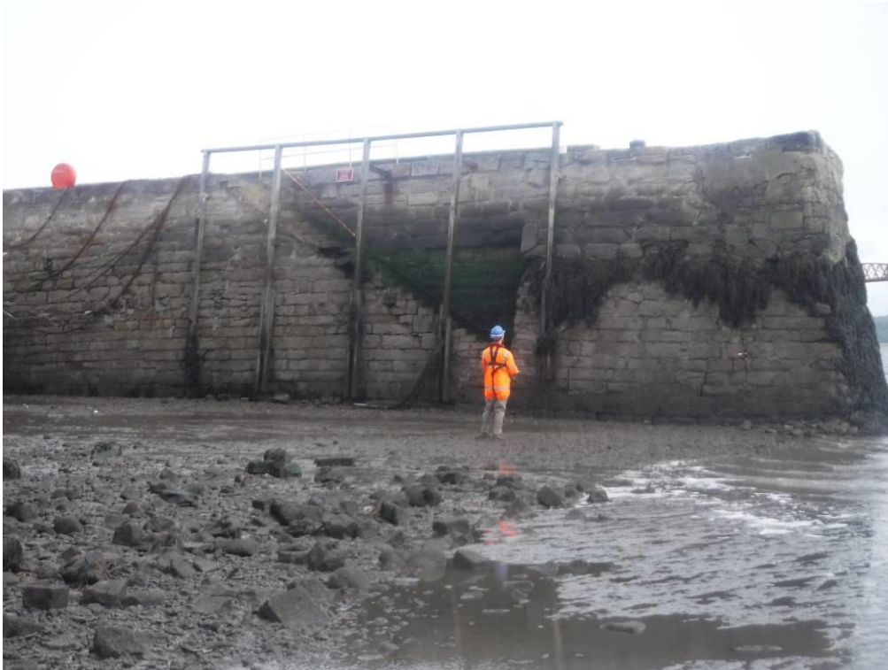
Photo 1 – View of north pier interior wall at harbour entrance. Note cracks, poor condition staircase, subsidence (in image LHS). Taken looking north.
