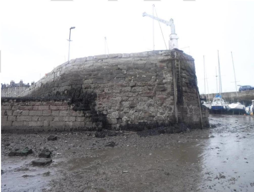
Photo 19 – Nose of eastern pier, taken looking south from harbour entrance. Note dilated joints/ full height cracking and possible bedrock exposed at base of structure. Metal davit on top of pier wall.
