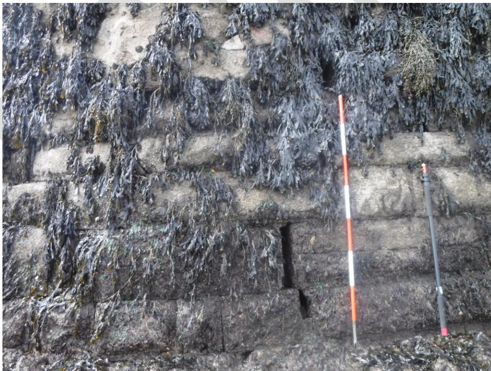
Photo 6 – View of typical voids/ dilated joints in outer wall of north pier, within approximately 20m of harbour entrance. Staff for scale is approximately 1600mm length, with 200mm gradations. Taken looking south from scour protection.
