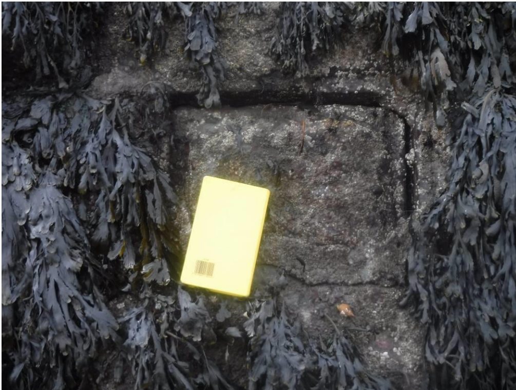
Photo 7 – Missing pointing around stone block, approximately 300 x 300mm. Yellow notebook for scale approximately 190mm long.
