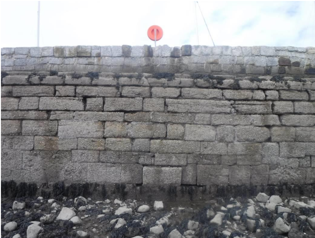
Photo 22 – Protruding block visible at toe of slipway wall in image centre front.. Note missing pointing and dilated joints in upper part of wall below cope stones, typical of slipway wall.
