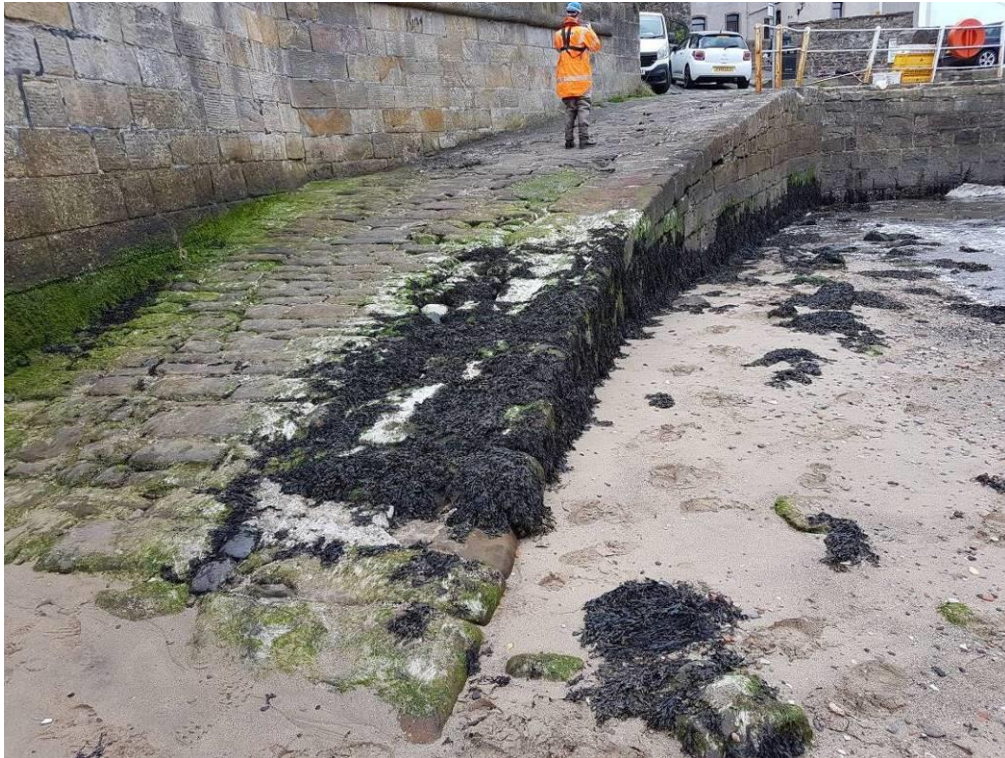
Photo 34 – View west of access ramp to eastern foreshore. Note distressed deck and semi-circular subsidence
