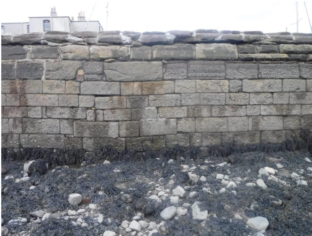
Photo 24 – Distressed/ misaligned stonework east slipway wall. Taken looking east, note dilated joints around upper courses.
