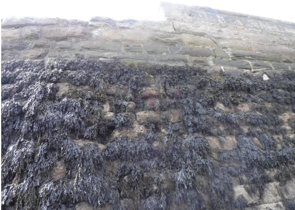
Photo 5 – View of weathered stonework within outer wall of north pier, partially obscured by seaweed. Note crack in right side of image extending from parapet wall, and weathered condition of stonework within tidal (seaweed) area. Located within 20.0m of harbour entrance.
