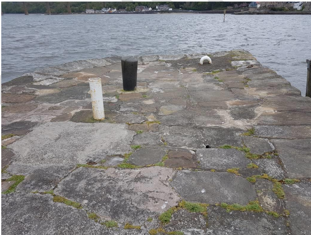
Photo 9 – View looking of subsidence area in deck of north pier, taken looking east along pier. Subsidence area measures approximately 8.0m x 5.0m. Note bollards out of vertical.
