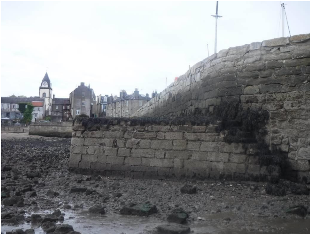
Photo 20 – View looking south at nose wall of east pier slipway. Note dilation in joints and cracking forming a wedge shaped block on corner with east facing wall of slip.
