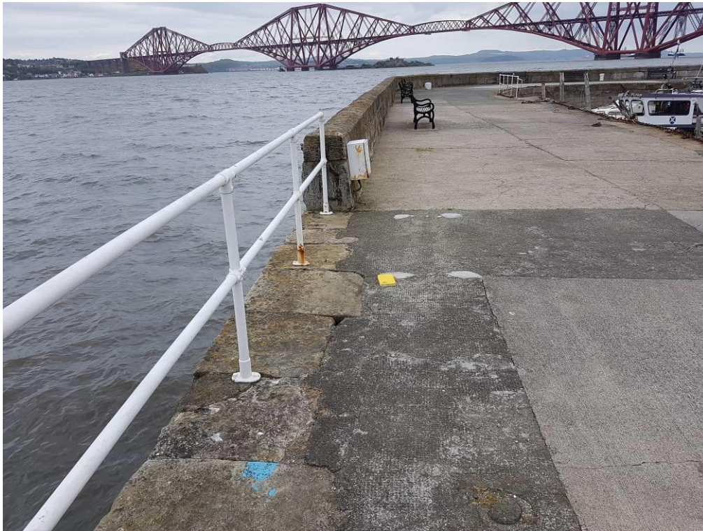
Photo 18 – Missing pointing around cope stone on outer wall of west pier, visible in surface to left of yellow notebook. Taken looking north along outside wall.
