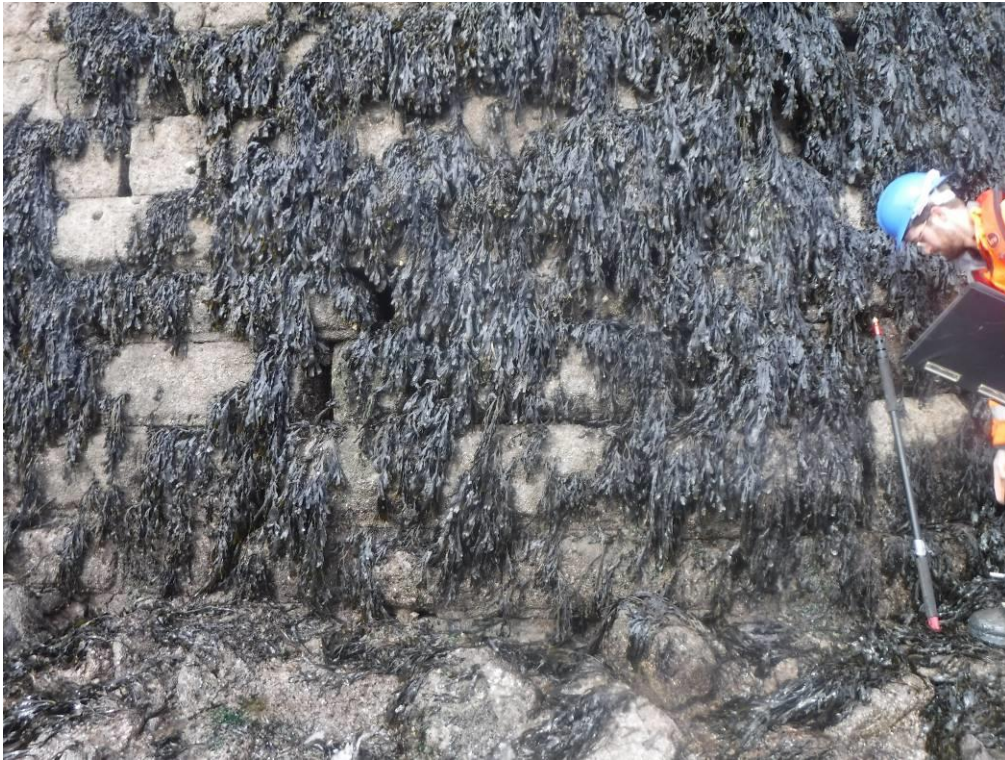
Photo 3 – Displaced blocks, dilated joints and voids within toe of north pier nose wall. Note crack defined block in image right fore, on corner of nose (east) and outer wall. Black staff for scale approximately 1.0m long.
