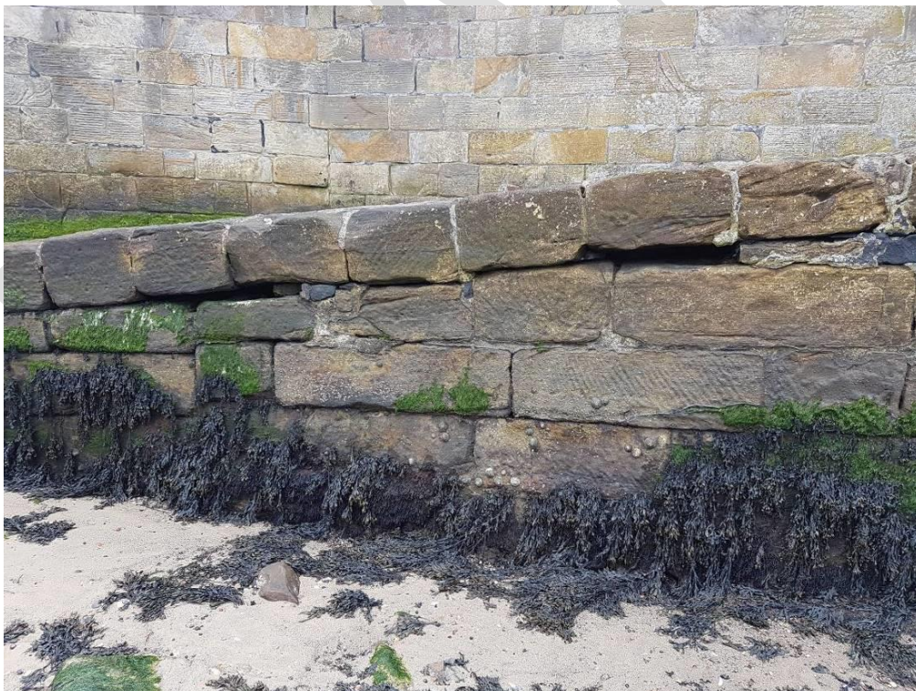
Photo 35 – View south of voids around cope stones in access ramp wall. Probed up to 800mm deep, congruent with area shown in Photo 34.
