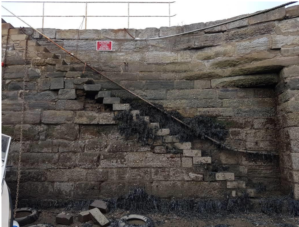
Photo 14 – View of staircase 1 (north) within inner wall of west pier. Note displaced/ missing stonework, missing mortar and poor condition rail. Displaced stonework visible on floor of harbour below staircase.
