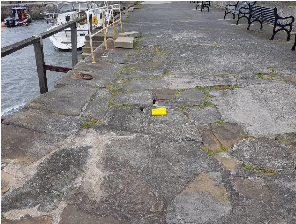
Photo 10 – View of void in mortar between stones blocks in deck of pier behind damaged staircase (north pier) taken looking west. Yellow notebook for scale approximately 200mm long. Void probed to approximately XXm.
