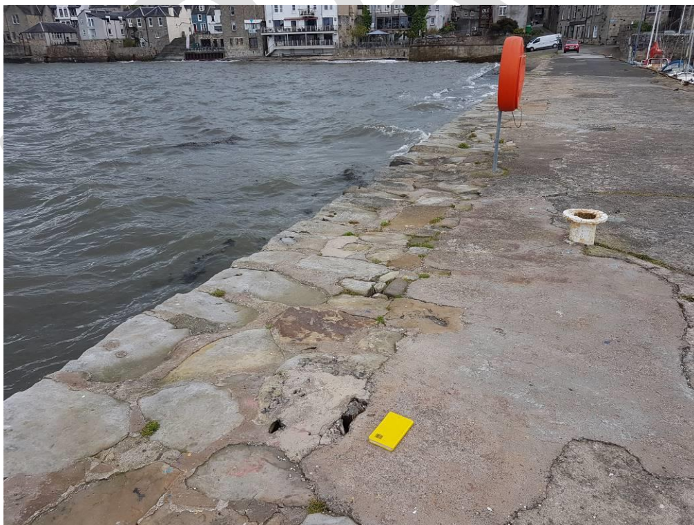
Photo 29 – View of east pier deck, approximately 10.0m south of harbour entrance. Void visible adjacent to yellow notebook (200mm length), probed to depth of XXXmm.
