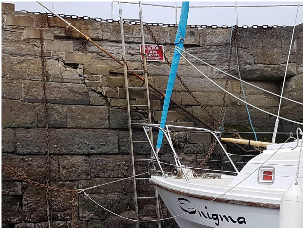
Photo 16 – Staircase 2 (middle) within west pier. Cracked lintel visible at head height. Note corroded hand rail, defective pointing and dilated/ displaced joints below cope stones.
