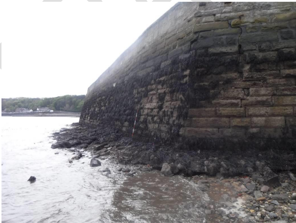
Photo 10 – View of void in mortar between stones blocks in deck of pier behind damaged staircase (north pier) taken looking west. Yellow notebook for scale approximately 200mm long. Void probed to approximately XXm.
