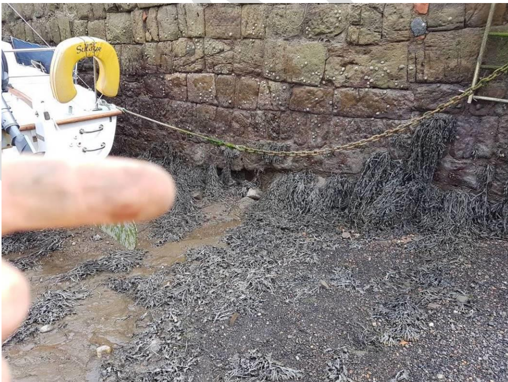
Photo 32 –Example of missing pointing and washed out historical repairs (voids) within interior wall of eastern pier.
