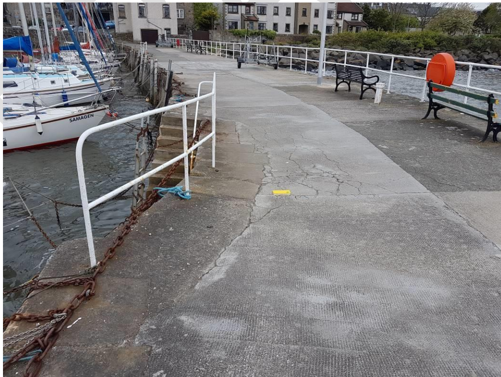
Photo 17 – Cracking and distress in concrete deck surfacing above Staircase 1, behind cope stones.
