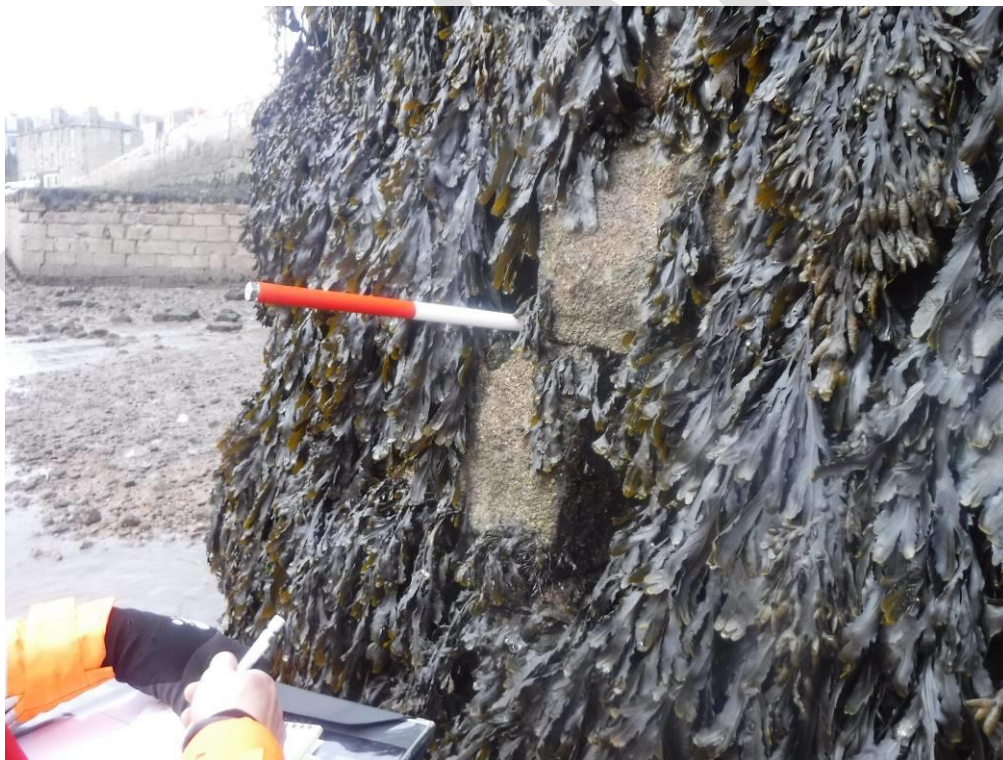
Photo 2 – View of typical dilated joints and voids between blocks visible within nose of north pier at harbour entrance. Staff for scale inserted into void up to 1200mm. Total staff length 1600mm. Taken looking approximately south west from nose, approximately 1.2m above ground level.
