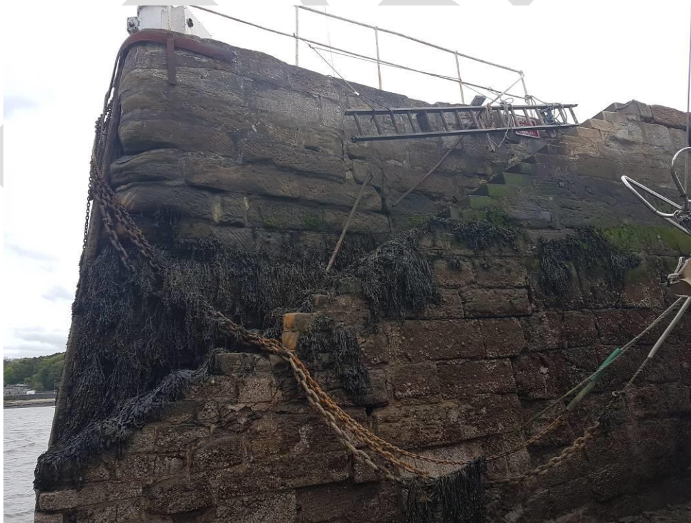
Photo 27 – View looking east of upper east pier interior wall. Poor condition staircase, distressed stonework, dilated joints visible. Corroded strapping visible on corner of wall in upper image left.
