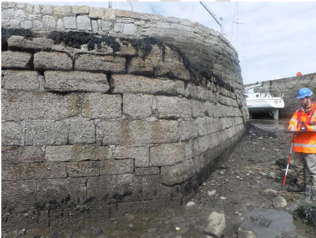
Photo 20 – View looking south at nose wall of east pier slipway. Note dilation in joints and cracking forming a wedge shaped block on corner with east facing wall of slip.
