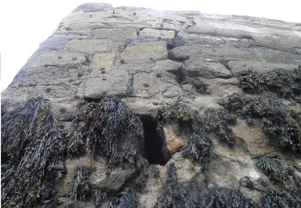
Photo 4 – View of dilated joints/ voids and defective pointing visible in upper part of north pier nose. Taken from toe of wall looking west at corner between nose and inner wall.
