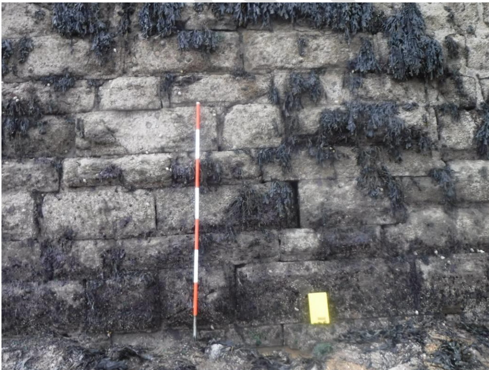
Photo 7 – Missing pointing around stone block, approximately 300 x 300mm. Yellow notebook for scale approximately 190mm long.
