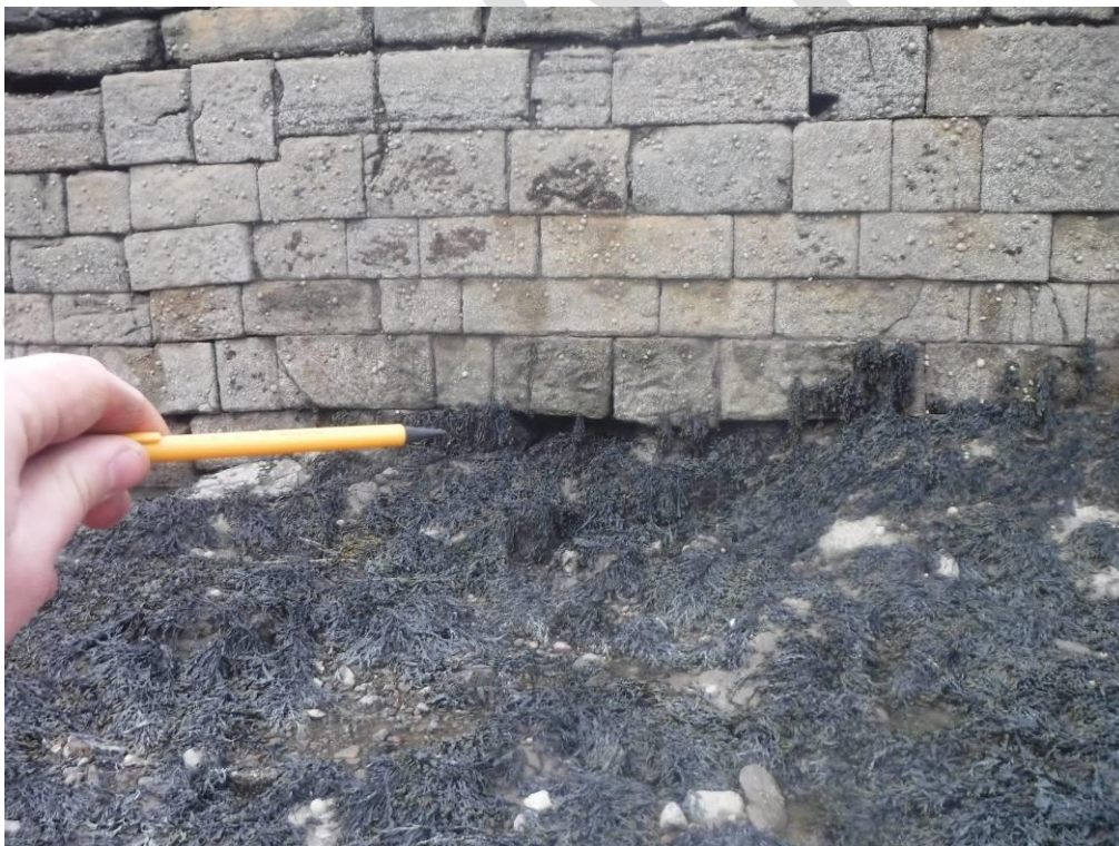
Photo 25 – Missing stone/ void at base of east slipway.
