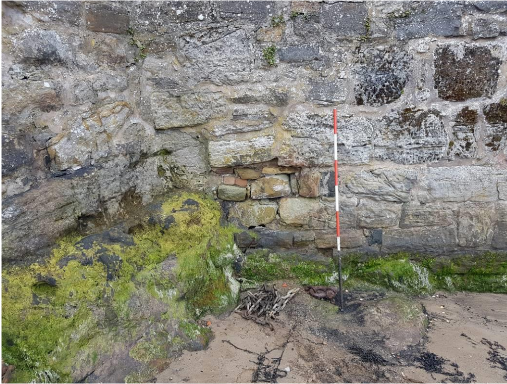
Photo 25 – Packed void at base of southern wall missing pointing. Staff for scale approximately 1.6m long with 0.2m gradations.
