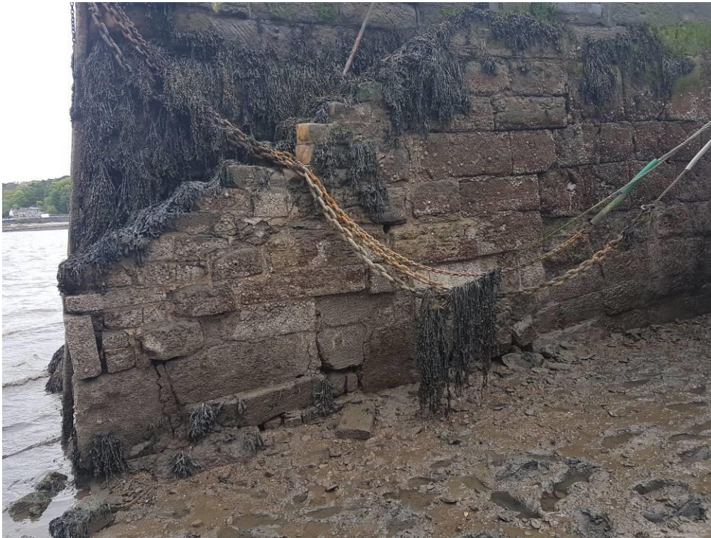
Photo 28 – Lower interior wall of east pier at harbour entrance. Note missing mortar, dilated joints and voids visible around blocks, displaced blocks also evident. Voids probed up to 1100mm depth.
