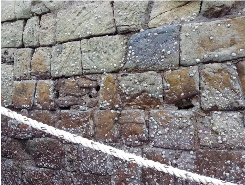
Photo 32 –Example of missing pointing and washed out historical repairs (voids) within interior wall of eastern pier.
