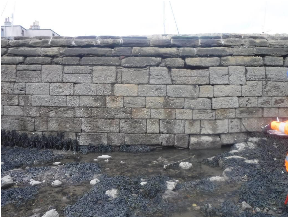
Photo 26 – Void and displaced stonework visible in water filled hollow at toe of slip wall. Note dilated joints and missing pointing in upper wall.
