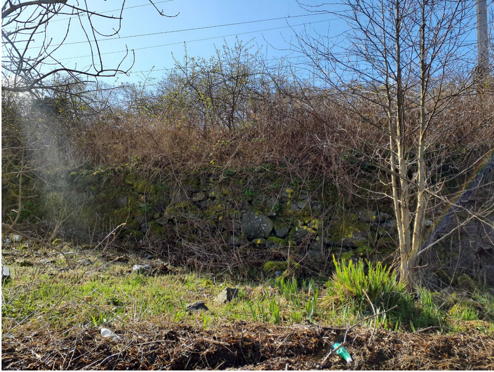
Western end of retaining wall
