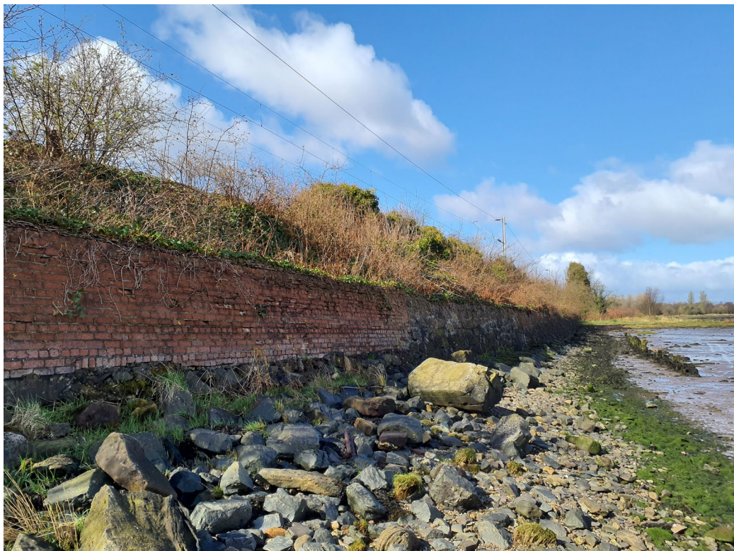
Close view of retaining wall looking westwards
