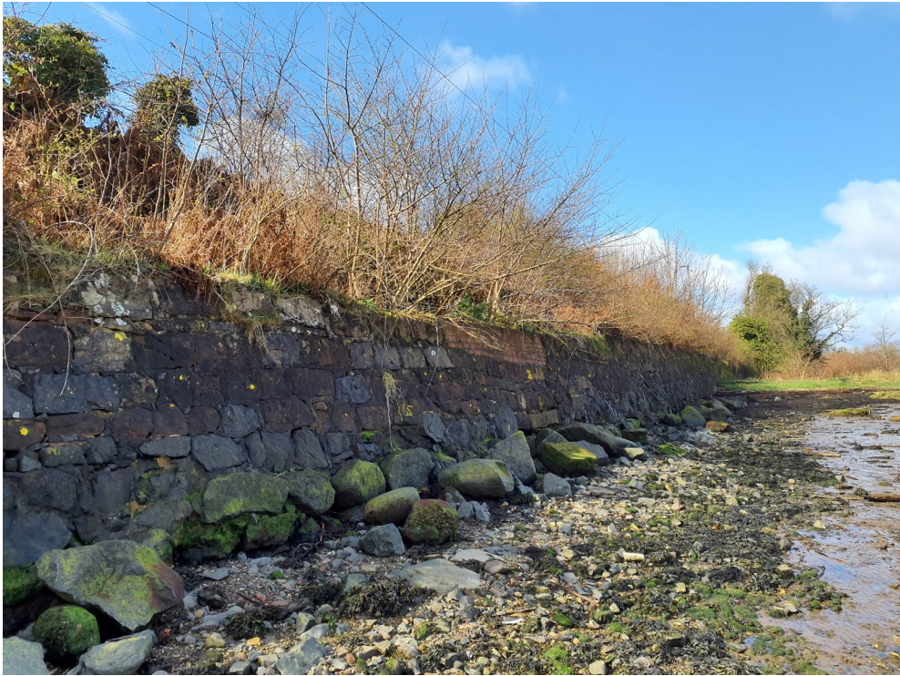
Eastern end of retaining wall looking westwards
