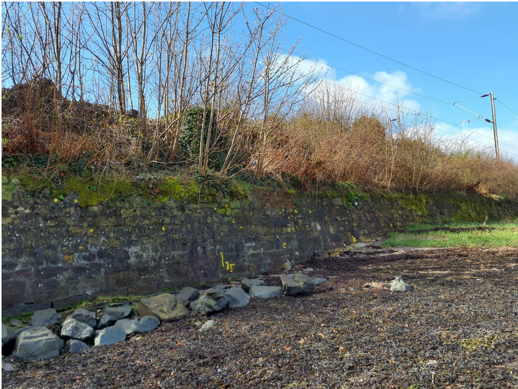
East end of retaining wall
