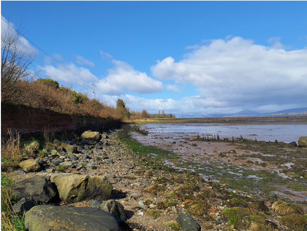
Overview of retaining wall and intertidal zone looking westwards
