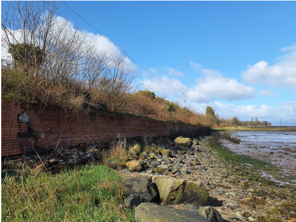
Overview of retaining wall looking westwards
