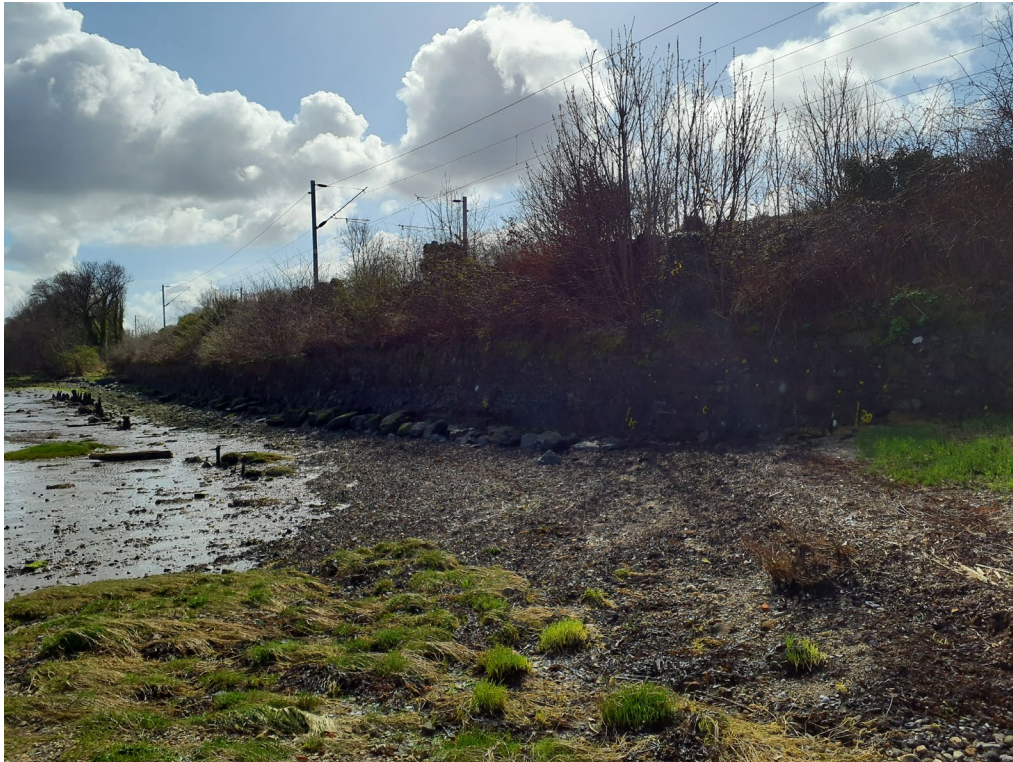
Eastern end of retaining wall looking eastwards
