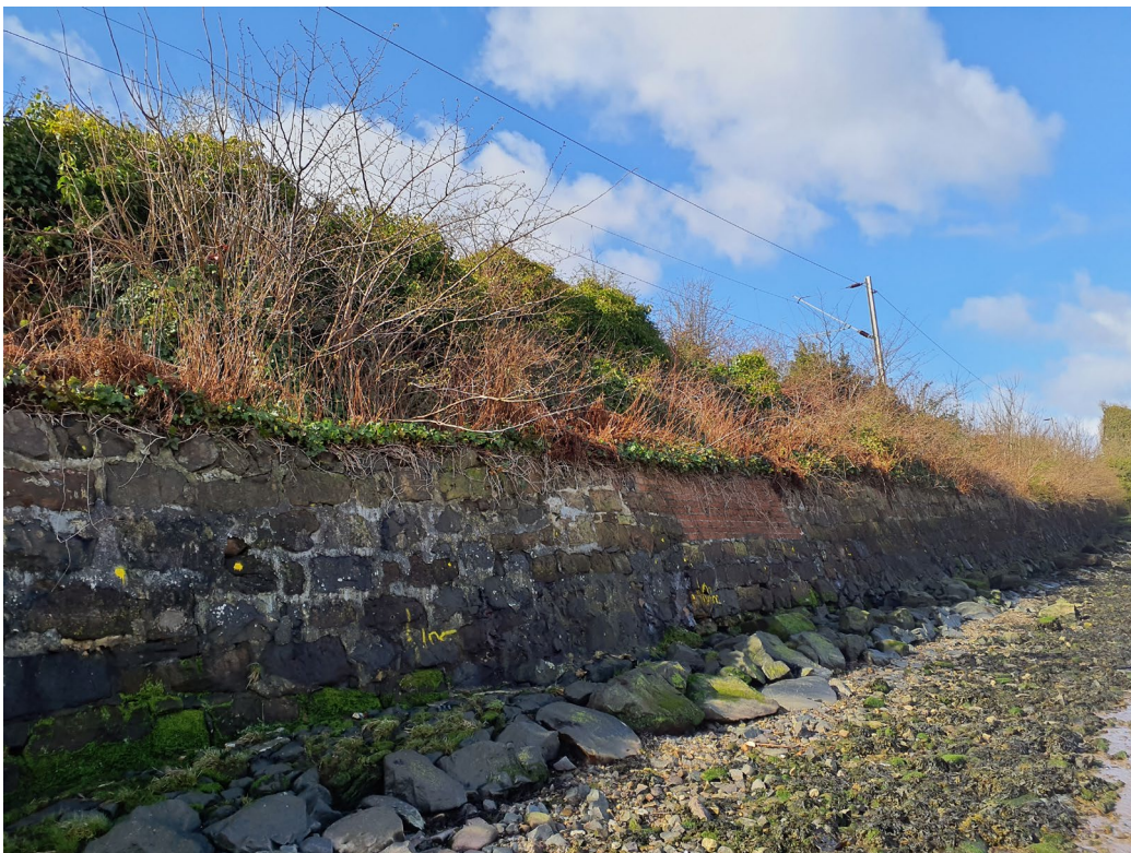
Mid to eastern section of retaining wall looking westwards
