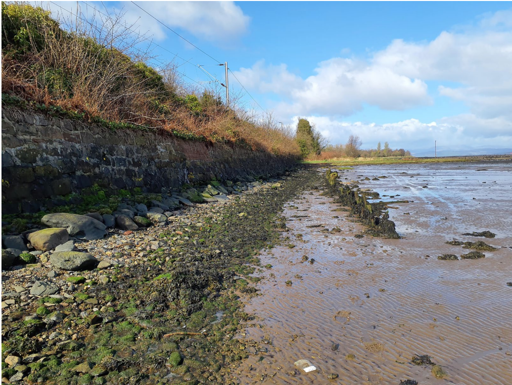
Approximate midpoint of retaining wall and intertidal zone looking westwards
