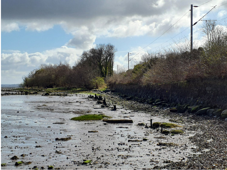
East end of retaining wall and intertidal zone looking eastwards
