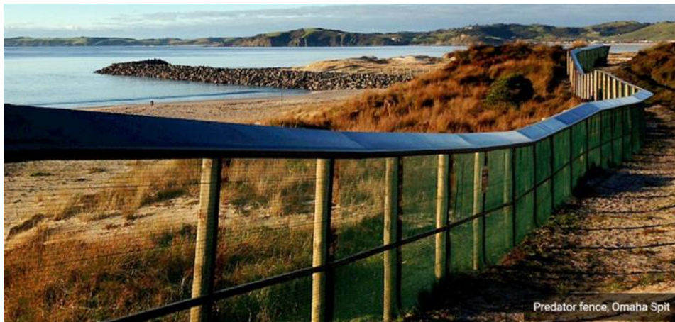
Figure 3-1 Example of a fence designed to exclude feral cats. The photograph shows a 375m long predator fence across Omaha Spit, north of Auckland for the Omaha Shorebird Protection Trust. The aim of the fence is to assist with predator management (including neighbouring domestic cats) so that shorebirds can nest on the ground.
