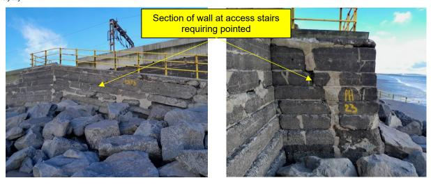
Utilising rope access equipment, sections of the wall displaying open joints will then be pointed. The wall will be pointed with a marine grade mortar. This will be flush pointed and brush finished.
