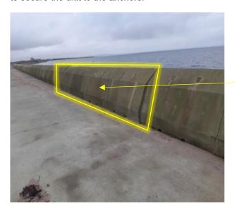
Section of four wave returns to be replaced
