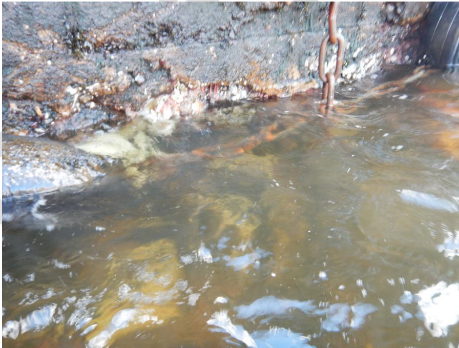
Photo 36 - Showing erosion to concrete below water line along berthing face
