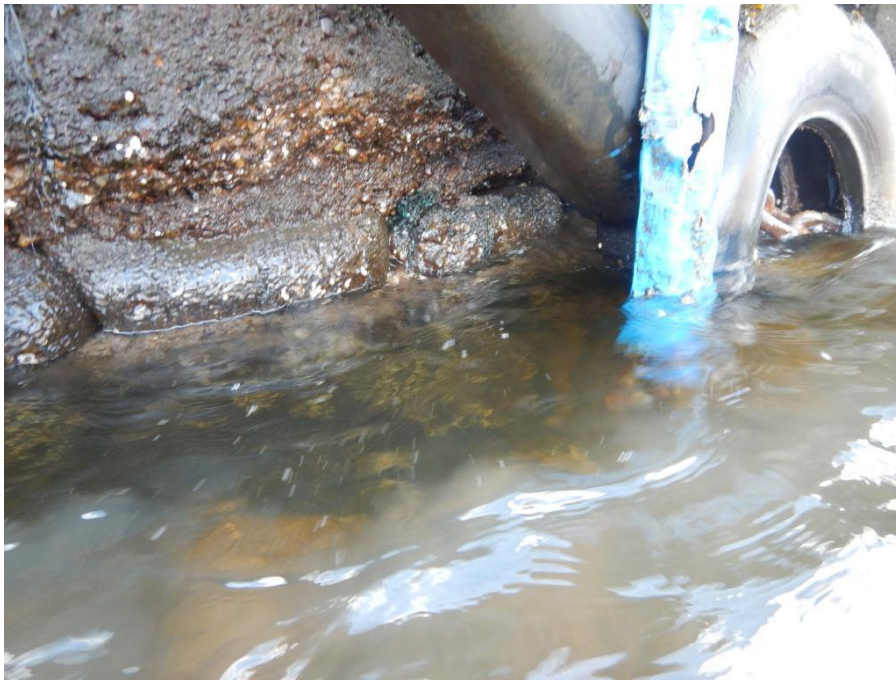
Photo 31 - Showing erosion to concrete below water line along berthing face
