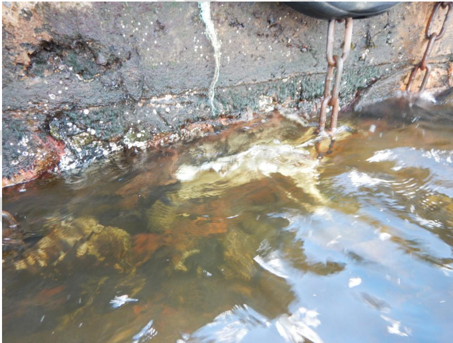
Photo 34 - Showing erosion to concrete below water line along berthing face
