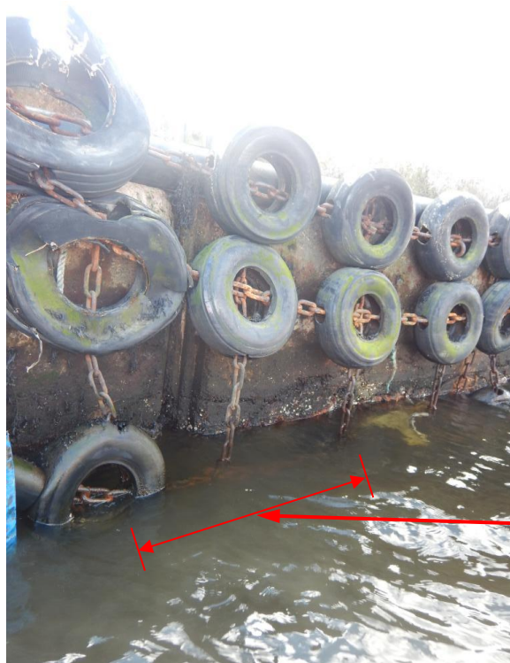
Photo 13 - Showing berthing face and fender arrangement with missing tyres along bottom chain
