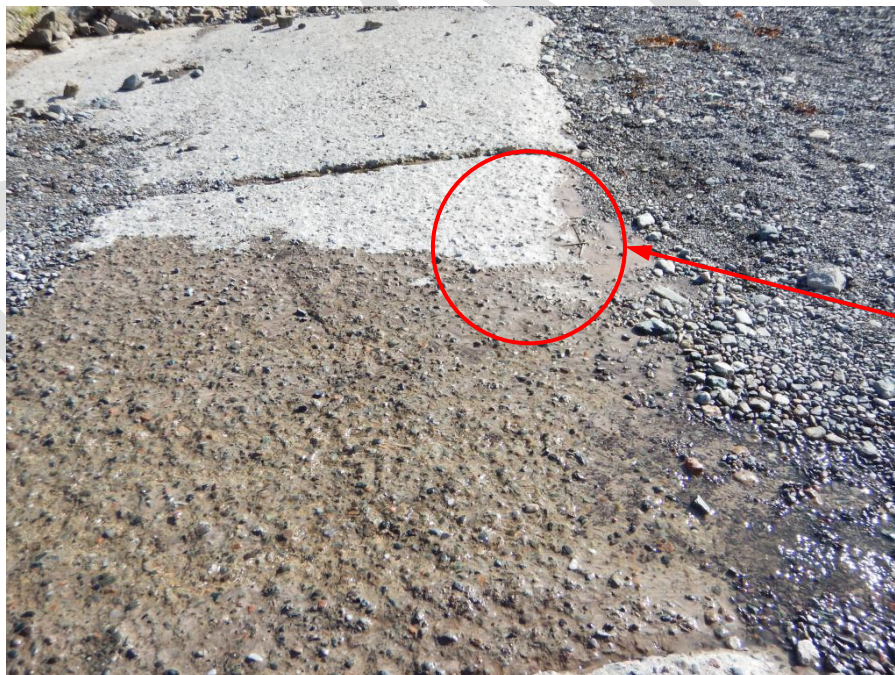
Photo 24 – Showing transition from informal surfacing to concrete transition slab
