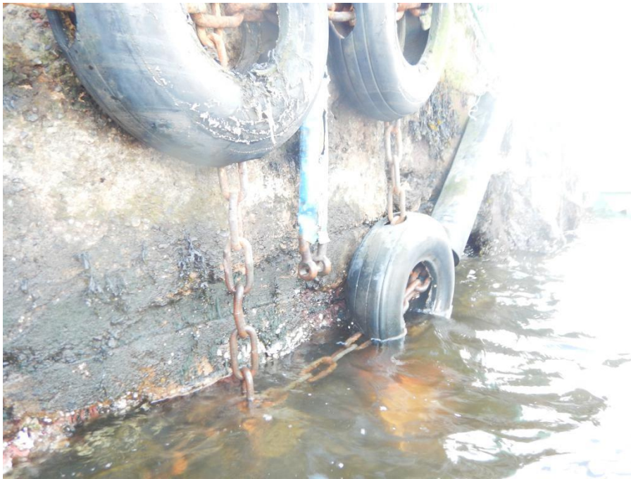
Photo 37 - Showing erosion to concrete below water line along berthing face
