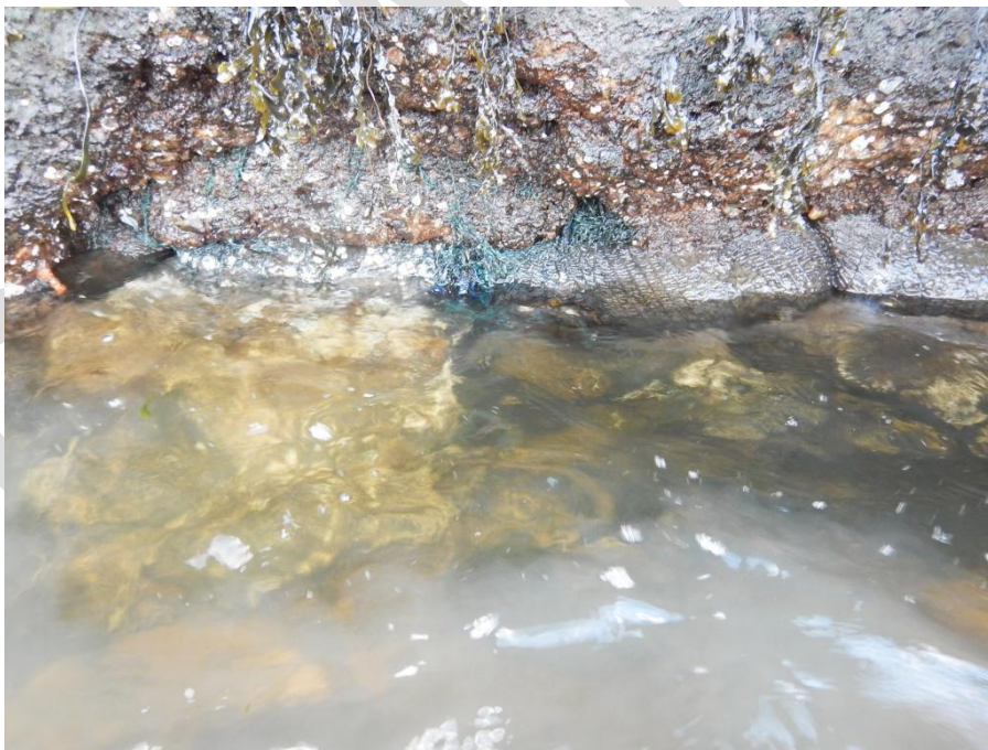
Photo 30 - Showing erosion to concrete below water line along berthing face
