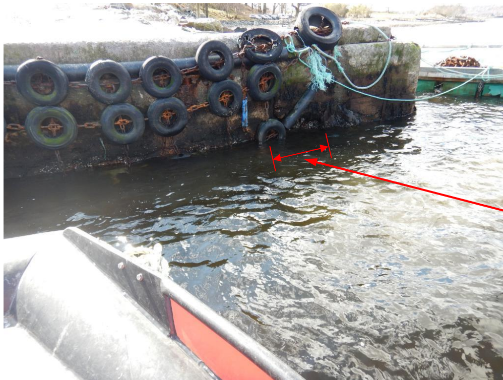
Photo 15 - Showing berthing face and fender arrangement with missing tyres along bottom chain
