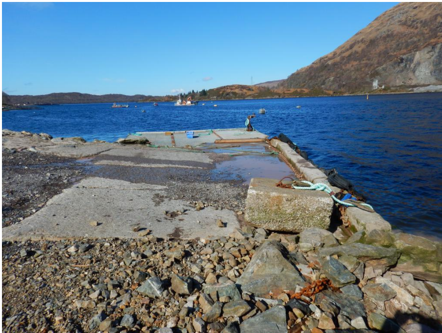
Photo 9 – Looking north west showing informal surfacing, concrete transition slabs and concrete pier
