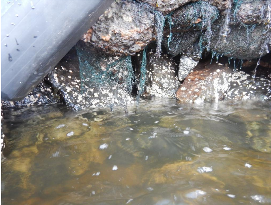
Photo 39 – Showing continuation of void
