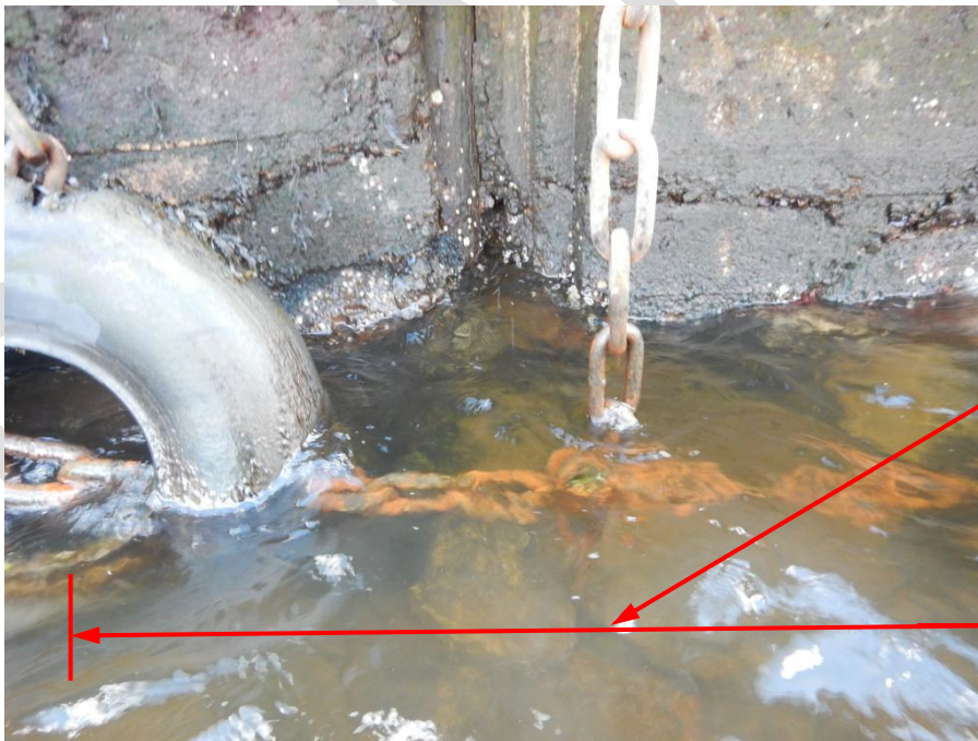
Photo 32 - Showing erosion to concrete below water line along berthing face
