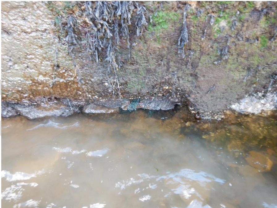
Photo 28 – Showing erosion to concrete below water line along berthing face starting at north east of pier
