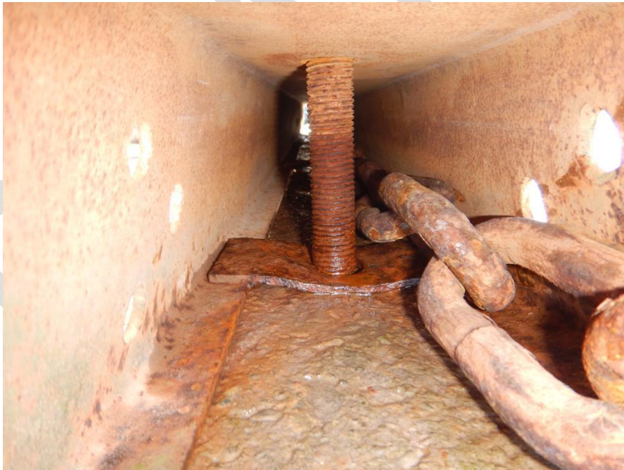
Photo 26 – Showing steel upstand securely fixed to concrete pier
