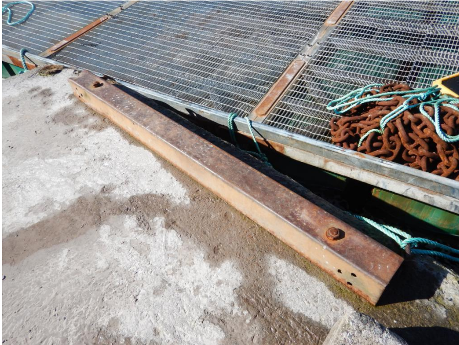
Photo 25 – Showing steel upstand
