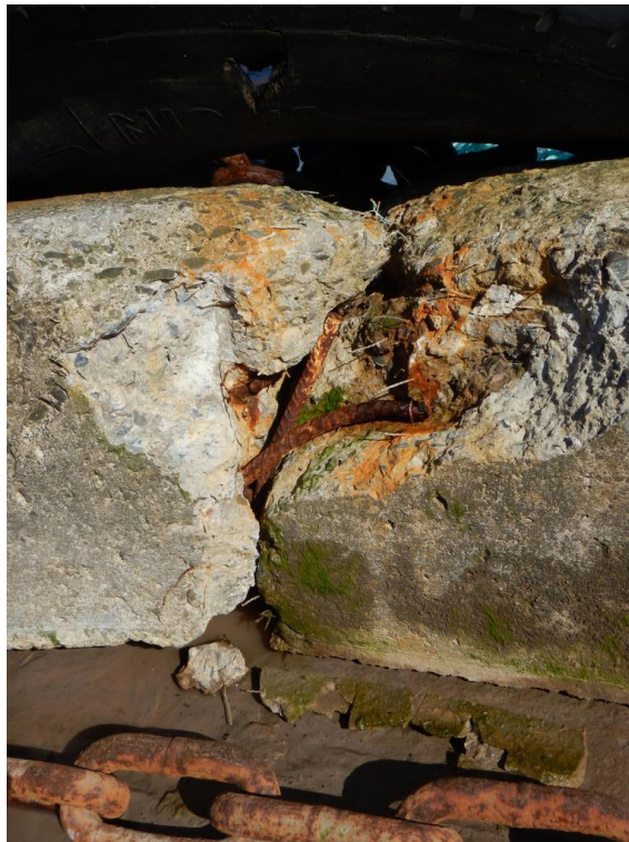
Photo 23 – Showing close up of damaged concrete upstand
