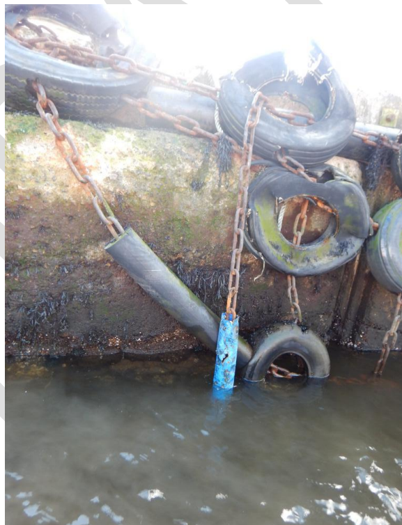
Photo 12 – Showing berthing face and fender arrangement
