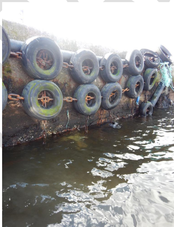
Photo 14 - Showing berthing face and fender arrangement with missing tyres along bottom chain
