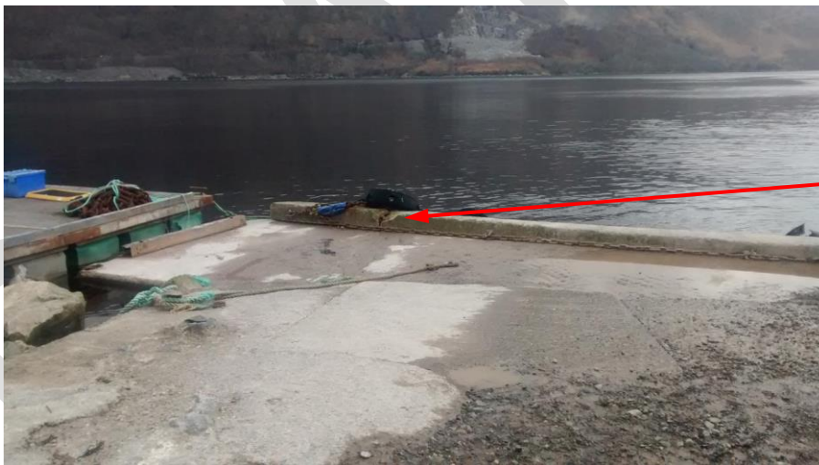
Photo 22 – Showing damaged concrete upstand
