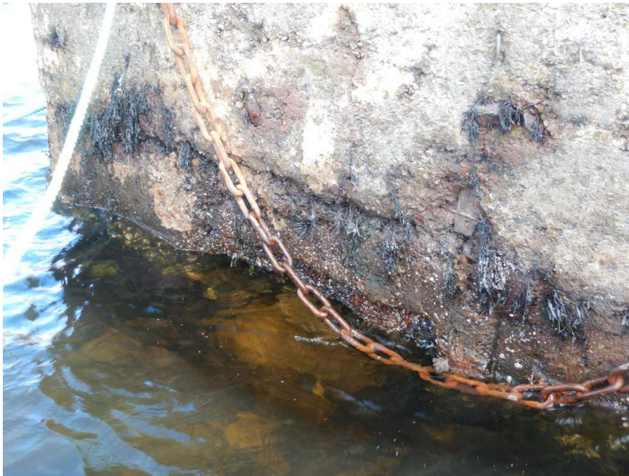
Photo 27 – Showing erosion below water line on north west return
