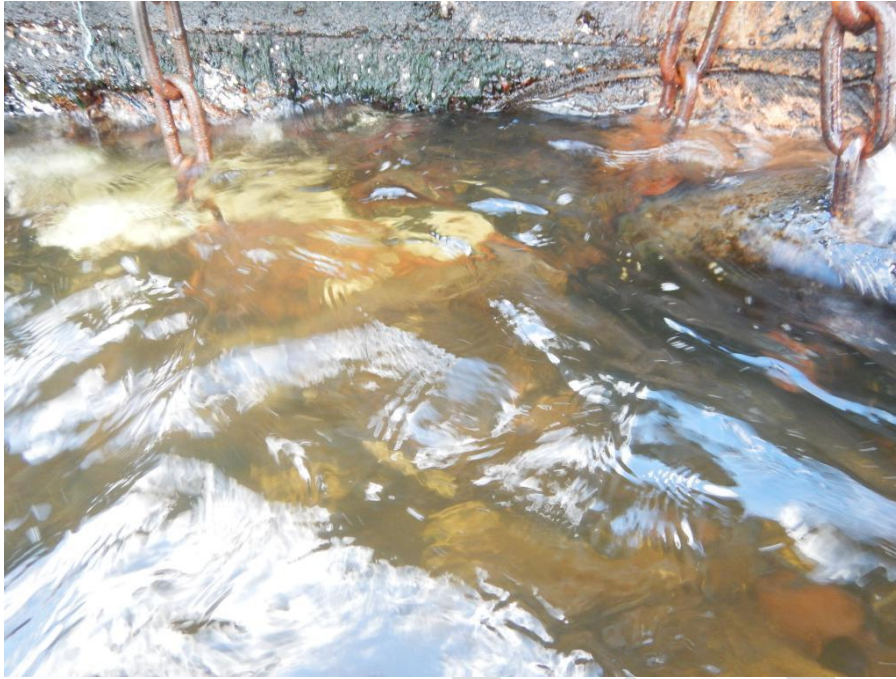
Photo 35 - Showing erosion to concrete below water line along berthing face
