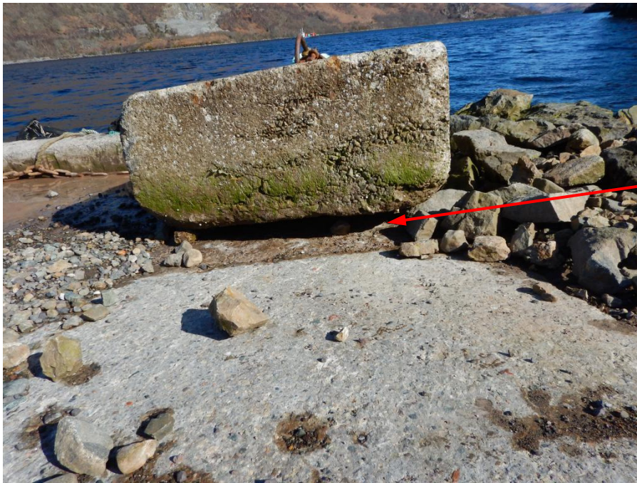
Photo 21 – Showing mass concrete block
