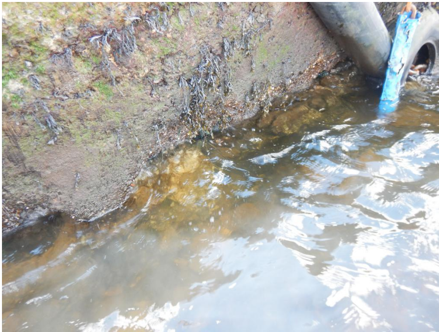
Photo 29 - Showing erosion to concrete below water line along berthing face
