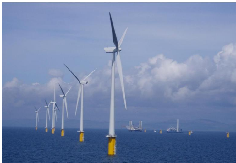
Figure 1.3: Photograph of Robin Rigg Offshore Wind Farm during the construction phase.
